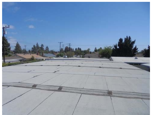
Photo #24: Portable classroom roof
