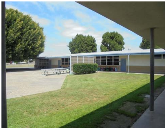
Photo #21: Courtyard between buildings
