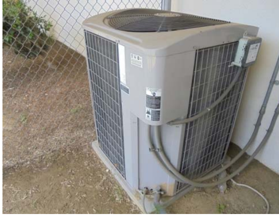
Photo #31: Condensing unit outside classroom
