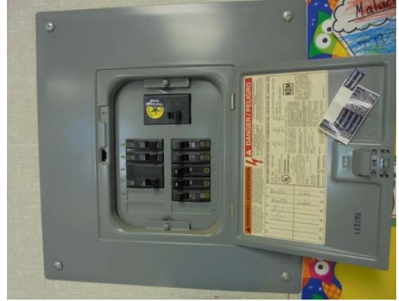
Photo #38: Electric panel in portable classroom
