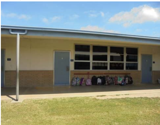
Photo #27: Classroom entrance windows and door
