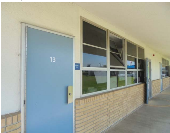
Photo #29: Awning windows at classrooms
