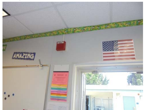
Photo #42: Fire alarm/strobe
