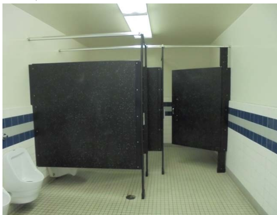
Photo #35: Renovated bathrooms
