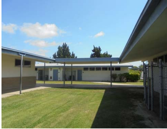
Photo #19: Covered walkway between buildings
