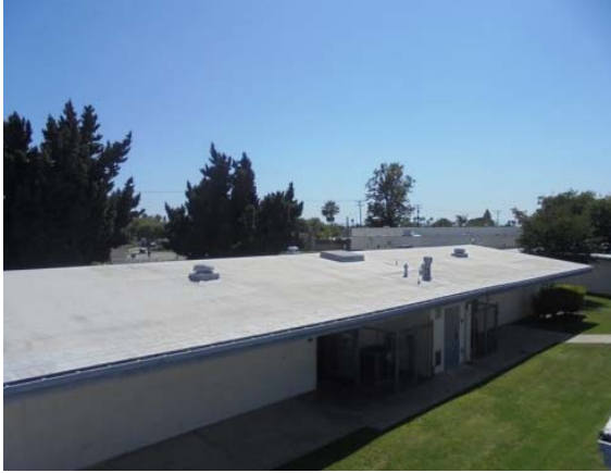
Photo #25: Classroom building roof
