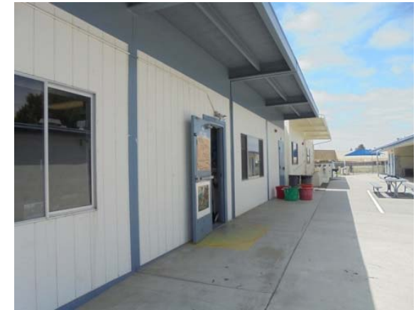
Photo #10: Portable classroom entrance
