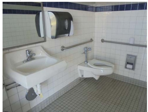
Photo #36: Renovated ADA bathroom
