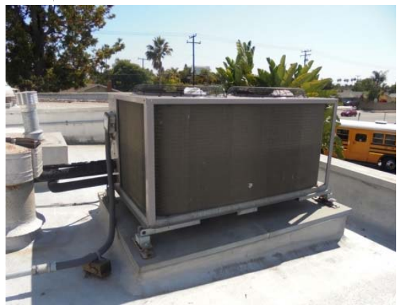
Photo #30: Roof top unit for Multi-purpose room
