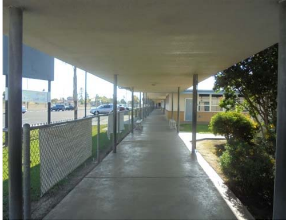
Photo #13: Covered walkways
