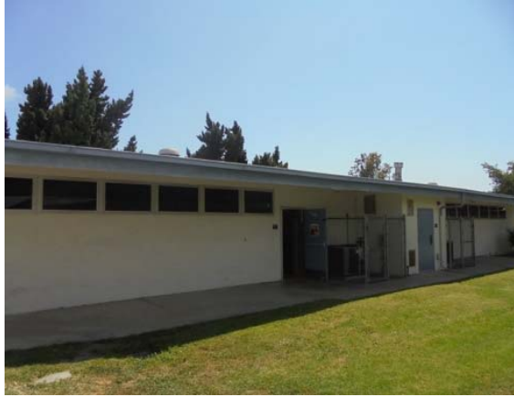
Photo #7: Rear elevation
