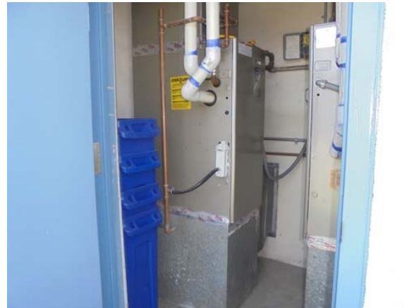
Photo #34: Classroom condensing furnace
