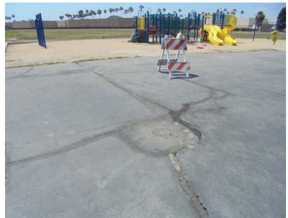
Photo #16: Damaged rear yard play surfaces
