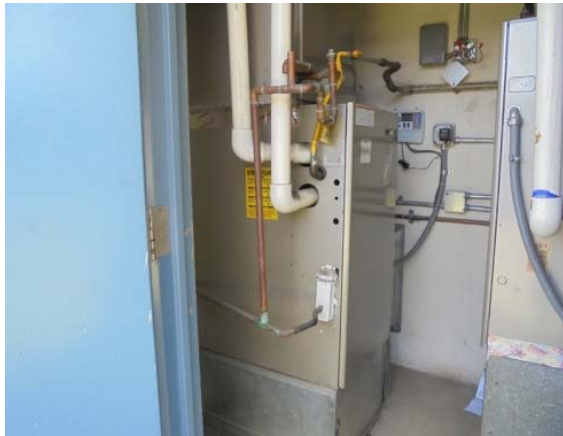
Photo #33: Classroom condensing furnace
