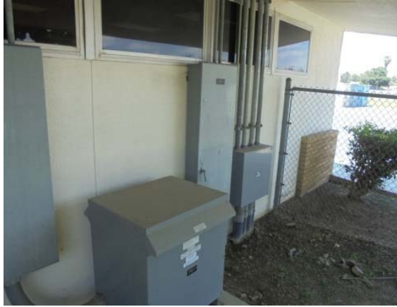
Photo #37: Transformer and electric panel
