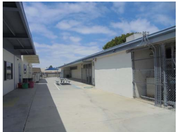
Photo #6: Rear elevation
