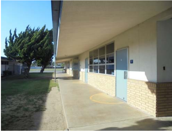
Photo #3: Classroom entrance
