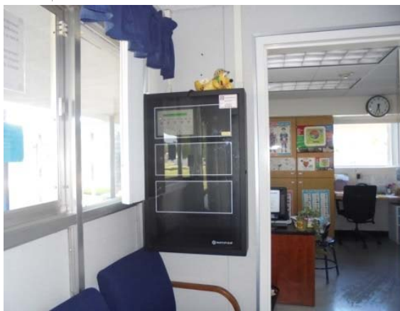
Photo #41: Fire alarm panel
