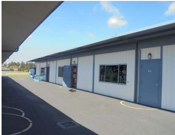
Photo #9: Portable classroom entrance
