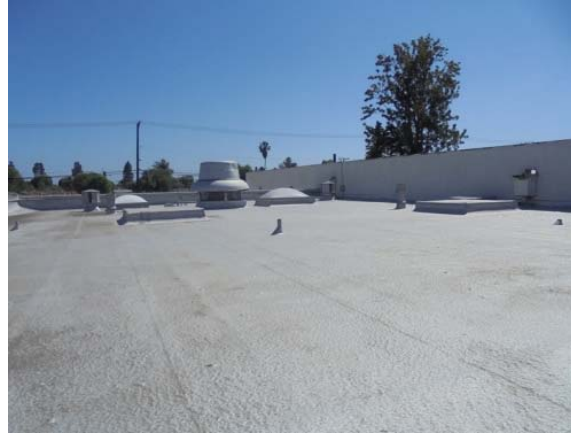
Photo #26: Multi-purpose building roof
