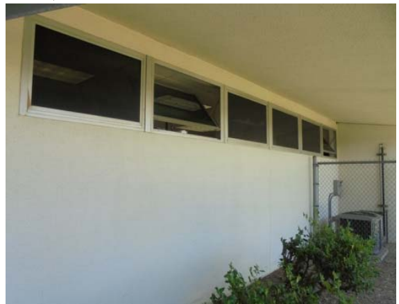
Photo #28: Rear elevation ribbon windows
