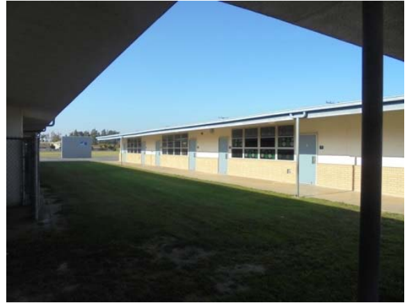
Photo #4: Classroom entrances
