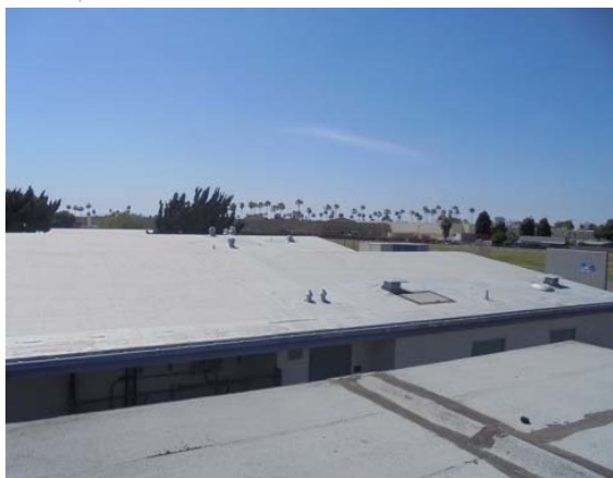
Photo #23: Classroom building roof
