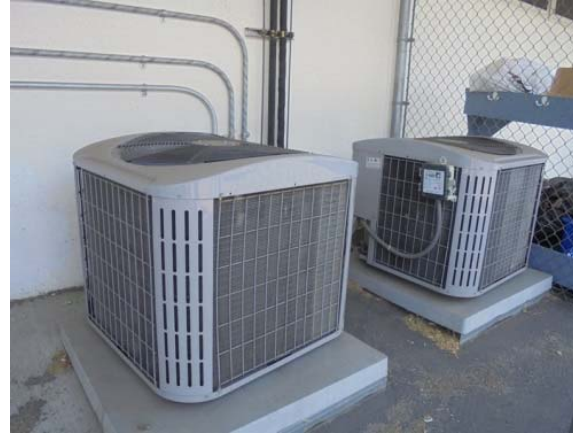
Photo #32: Condensing units outside of classrooms
