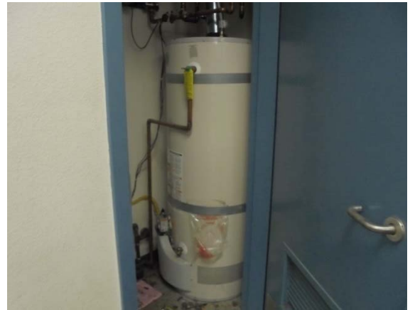
Photo #34: Water Heater at Gymnasium
