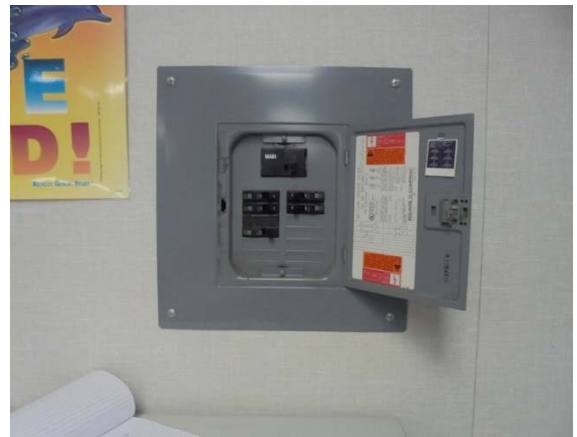
Photo #36: Portable Classroom Electric Panel
