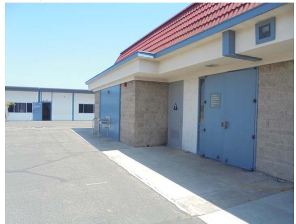
Photo #22: Multi-Purpose Room and Restrooms Entry Doors
