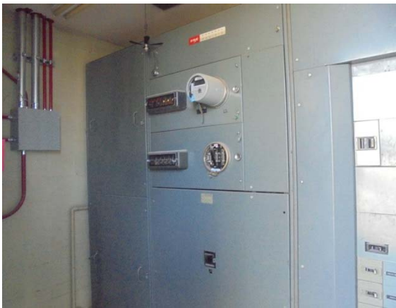
Photo #35: Main Electric Service at Main Building
