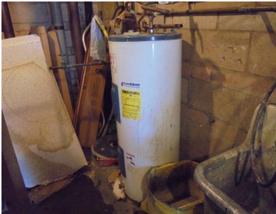
Photo #33: Water Heater at Main Building
