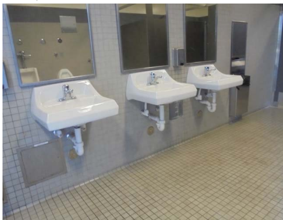
Photo #41: Central Restrooms at Main Building
