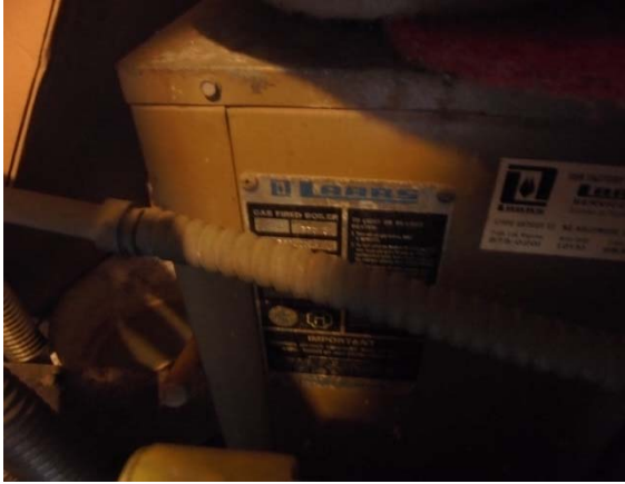
Photo #31: Abandoned Boiler at Main Building
