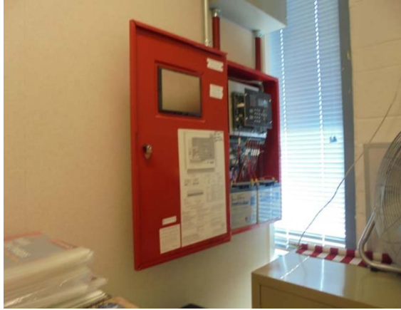
Photo #37: Fire Alarm Panel at Main Building
