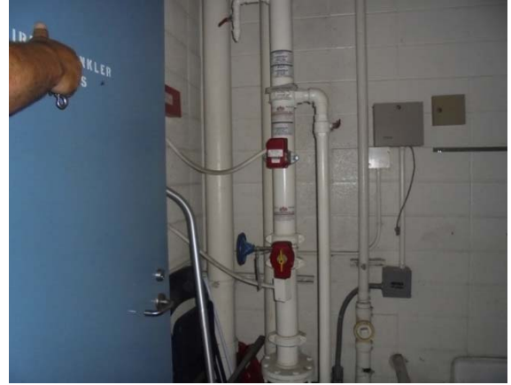
Photo #38: Standpipe at Gymnasium Building
