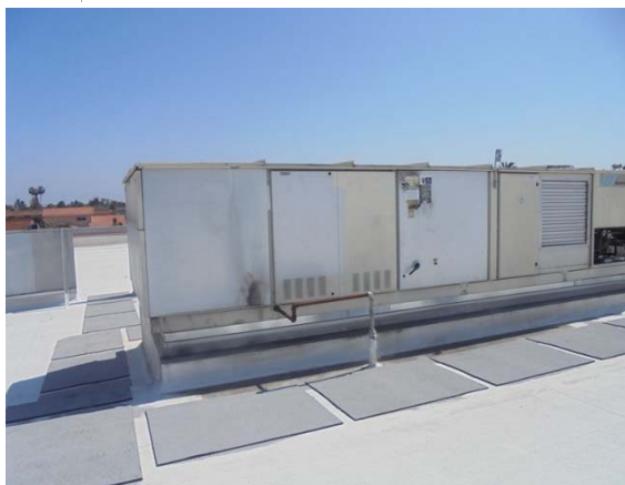
Photo #23: Roof Top Units
