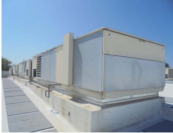
Photo #25: Roof Top Unit at Main Building
