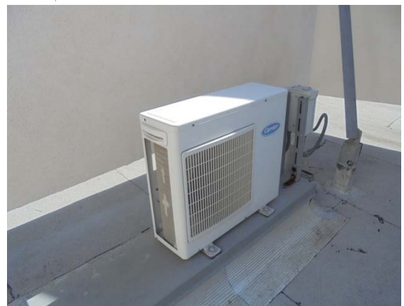
Photo #30: Split System for Offices/Classroom at Gymnasium
