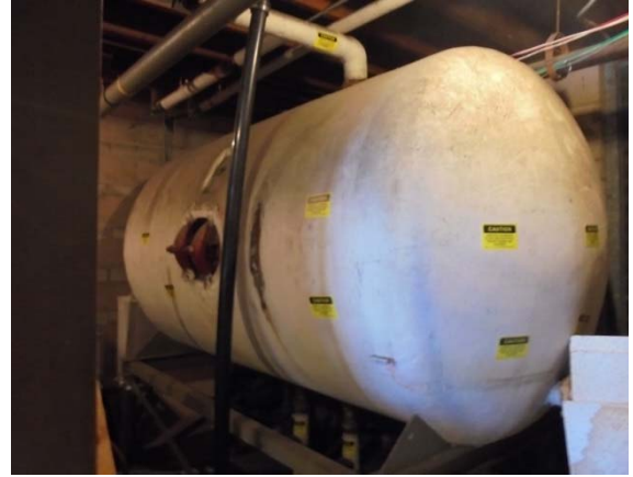
Photo #32: Abandoned Water Storage Tank
