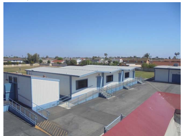
Photo #6: Portable Classrooms With Restrooms Wing
