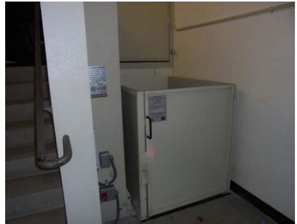
Photo #40: Wheelchair Lift at Gymnasium
