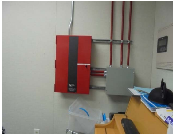
Photo #39: Sub-Panel for Portable Classrooms
