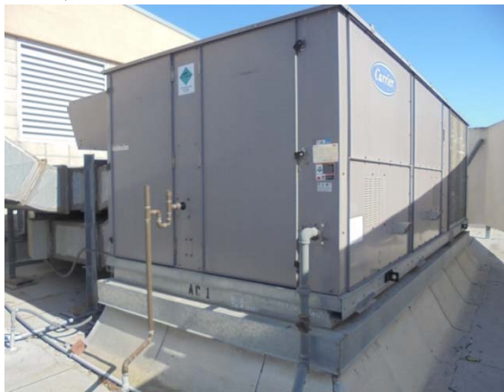
Photo #27: Roof Top Unit for Gymnasium
