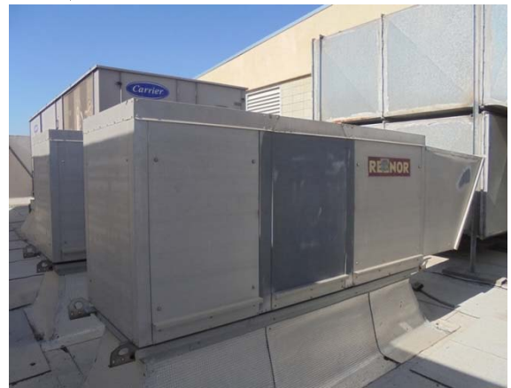
Photo #28: Heating Unit for Locker Room
