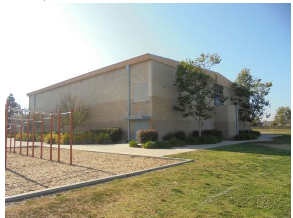
Photo #4: Rear Elevation Gymnasium
