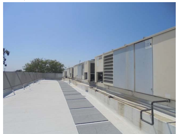
Photo #24: Roof Top Unit at Main Building
