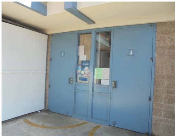
Photo #21: Classroom Entrance Doors and Windows
