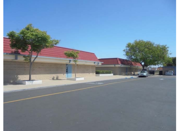
Photo #8: Main Building Front Elevation
