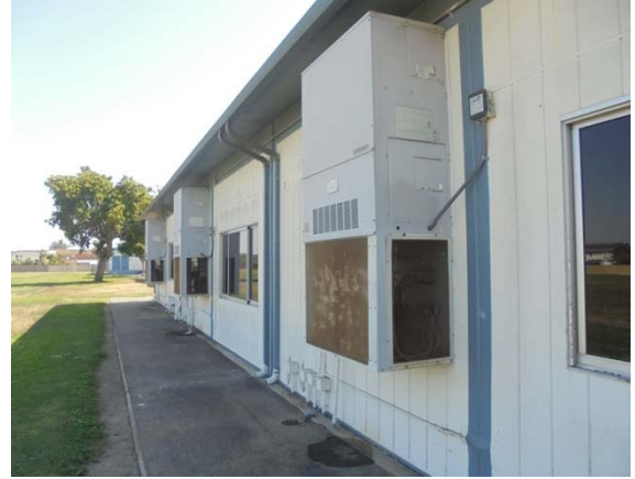
Photo #26: Heat Pumps at Portable Classrooms
