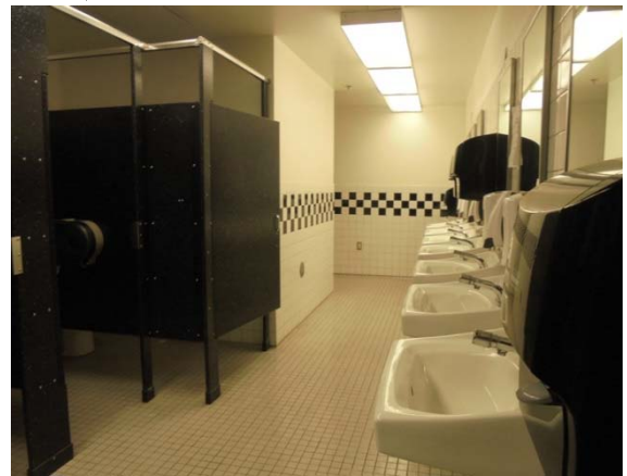
Photo #46: Restrooms At Gymnasium
