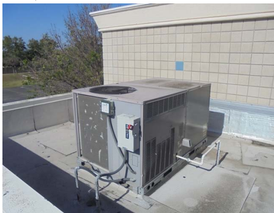
Photo #29: Roof Top Unit at Main Building
