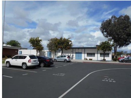
Photo #4: West Elevation
