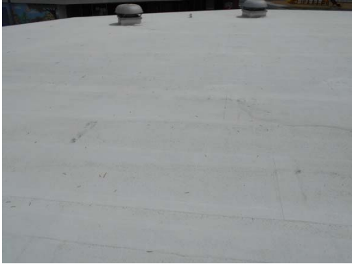
Photo #19: Classroom Pod Built-up Roof
