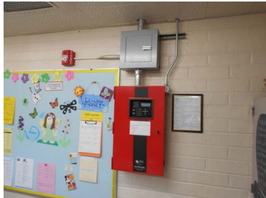
Photo #40: Central Fire Control Panel in Main Office
