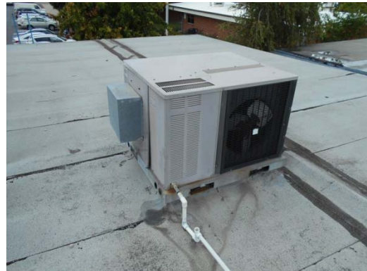
Photo #34: Heat Pump Unit at Portable Building
