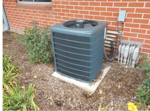
Photo #32: Condensing Unit at Office Building
