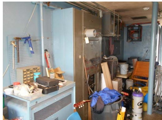
Photo #36: Electric Switchgear
