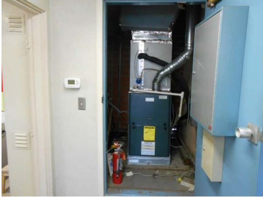
Photo #31: Furnace at Office Building
