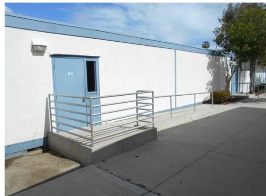
Photo #30: Concrete Ramp in front of Entrance
