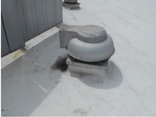
Photo #37: Powered Roof Vent
