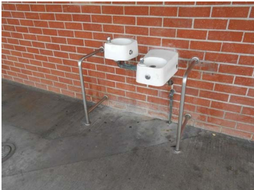
Photo #15: Drinking Fountains at Exterior of Building
