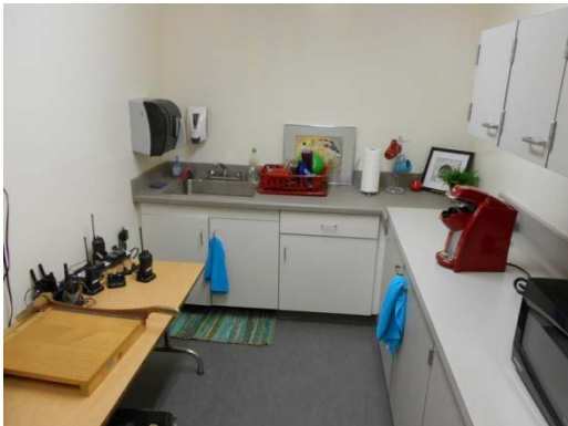
Photo #51: Casework in Office
