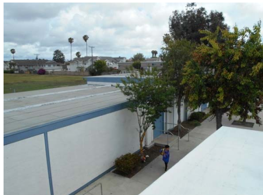
Photo #24: Painted Wood Siding
