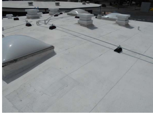
Photo #20: Restroom / Food Service Building Built-up Roof
