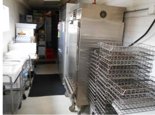
Photo #44: Reach-in Refrigerator
