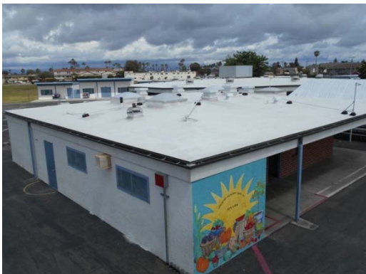
Photo #23: Stucco Walls
