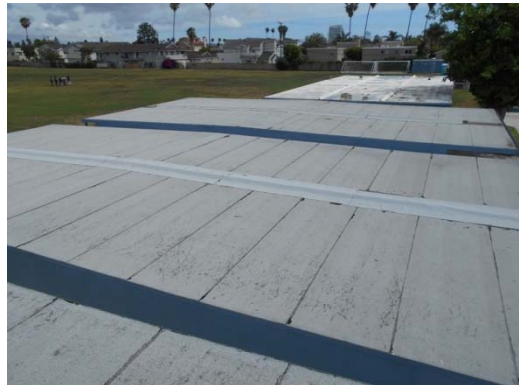
Photo #22: Portable Building Built-up Roof
