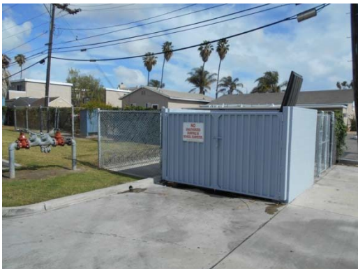
Photo #17: Trash Dumpster Enclosure
