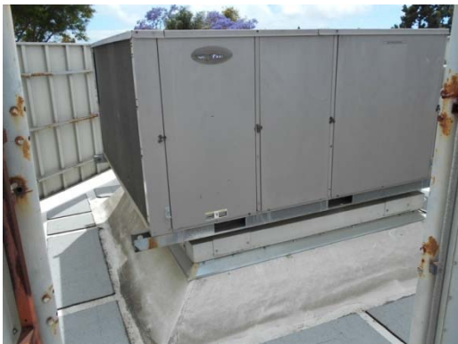
Photo #35: Heat Pump Package Unit at Classroom Pod
