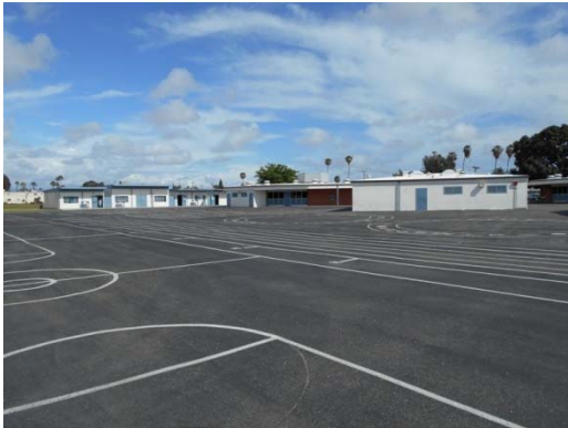
Photo #3: Northwest Elevation
