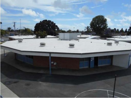
Photo #25: Classroom Pod Brick Walls
