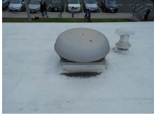
Photo #38: Gravity Roof Vent
