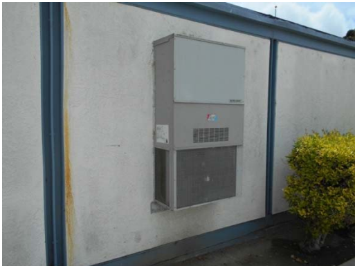
Photo #33: Heat Pump Unit at Portable Building
