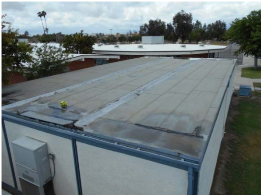
Photo #21: Portable Building Built-up Roof
