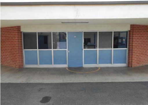
Photo #27: Classroom Pod Entrance
