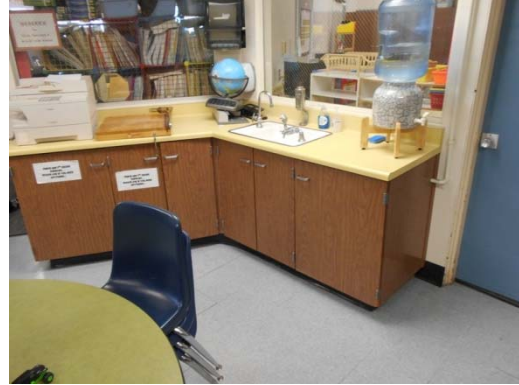
Photo #50: Casework in Classroom
