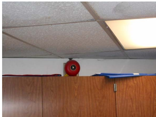
Photo #42: Alarm Bell
