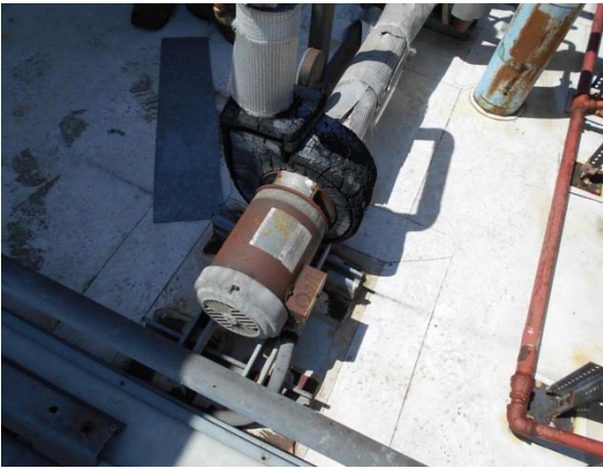
Photo #33: Water Circulating Pump
