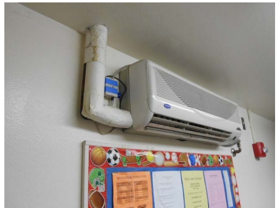
Photo #36: Ductless Split Air Conditioning Unit
