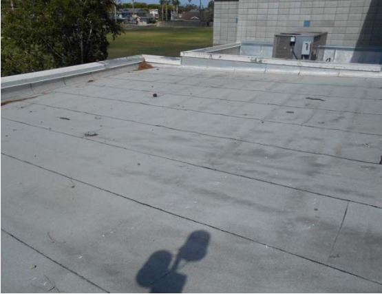
Photo #19: Buildup Roof at Gymnasium Building
