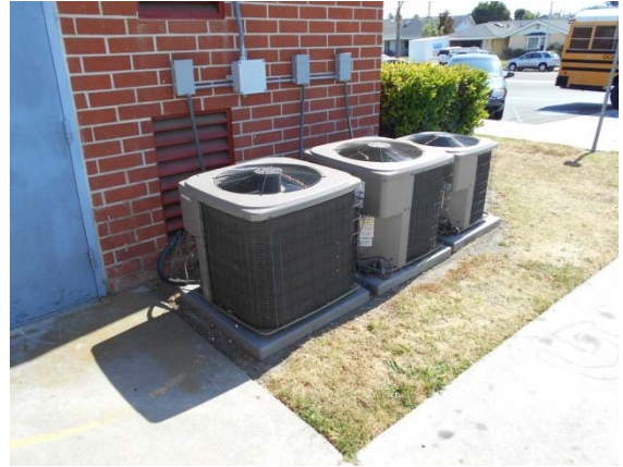
Photo #38: Condensing Units
