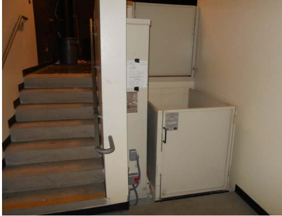
Photo #49: Gym Stage Wheelchair Lift
