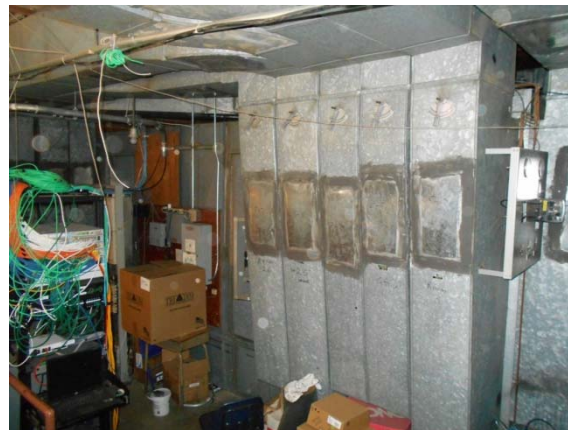
Photo #30: Interior Air Handling Units
