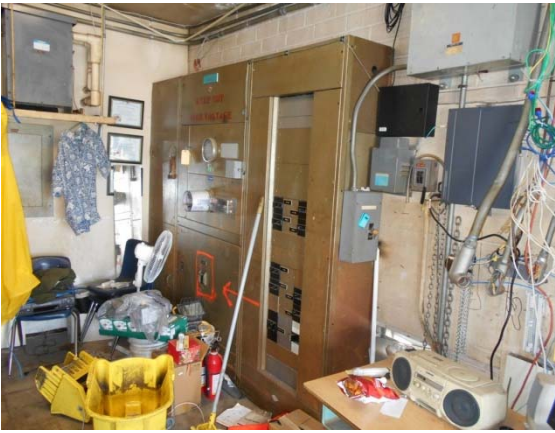
Photo #27: Main Electric Switchgear
