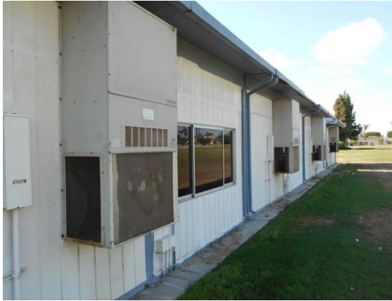
Photo #37: Wall Mounted Heat Pump
