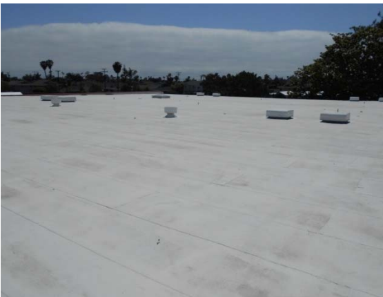
Photo #17: Main Classroom Building Built-up Roof
