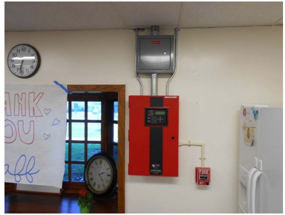
Photo #28: Central Fire Alarm Panel
