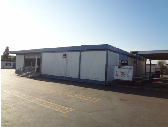
PHOTO #7: 4 CLASSROOM BUILDING ELEVATION
