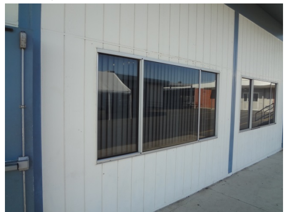
PHOTO #24: PORTABLE BUILDING SLIDING TYPE WINDOW
