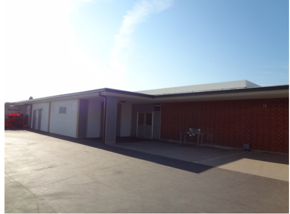
PHOTO #2: MAIN BUILDING LEFT ELEVATION
