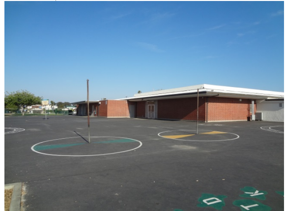
PHOTO #4: MAIN BUILDING RIGHT ELEVATION
