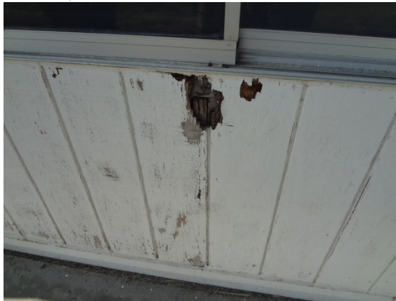
PHOTO #21: PORTABLE BUILDING DAMAGED WOOD SIDING
