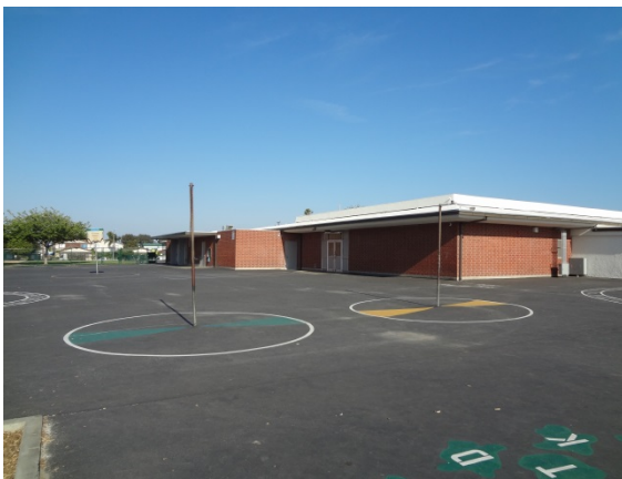
PHOTO #11: ASPHALT STUDENT PLAYGROUND
