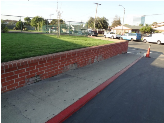
PHOTO #15: BRICK RETAINING WALL MAIN ENTRANCE
