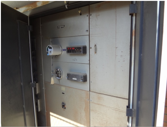
PHOTO #27: MAIN BUILDING SWITCHGEAR
