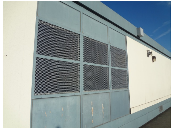
PHOTO #22: 4-CLASSROOM BUILDING STUCCO FAÇADE
