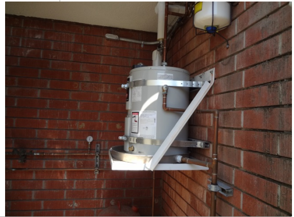
PHOTO #28: ELECTRIC WATER HEATER
