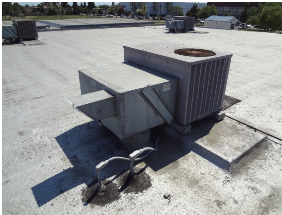
PHOTO #29: ROOFTOP HEAT PUMP
