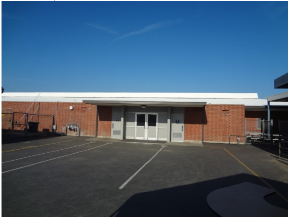
PHOTO #3: MAIN BUILDING REAR ELEVATION
