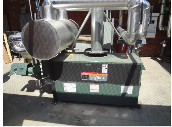
PHOTO #26: MAIN BUILDING GAS BOILER
