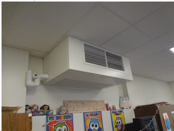
PHOTO #33: MAIN BUILDING 4-PIPE FAN COIL UNIT
