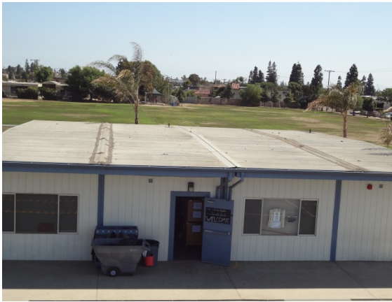
PHOTO #5: TYPICAL PORTABLE CLASSROOM FRONT ELEVATION
