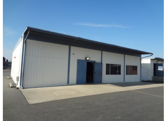
PHOTO #20: PORTABLE BUILDING ENGINEERED WOOD FAÇADE
