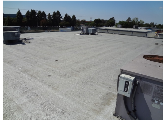
PHOTO #16: TYPICAL ASPHALT MEMBRANE ROOF
