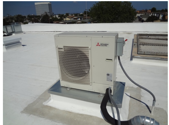
PHOTO #30: MAIN BUILDING COMPUTER ROOM DUCTLESS SPLIT SYSTEM
