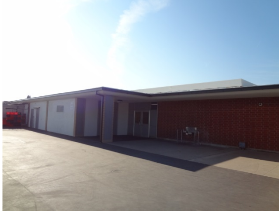
PHOTO #19: MAIN BUILDING BRICK VENEER FAÇADE
