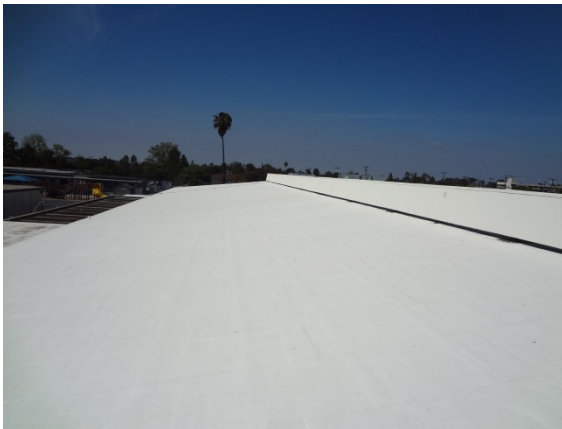
PHOTO #17: MAIN BUILDING NEW ASPHALT MEMBRANE ROOF
