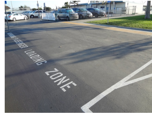
PHOTO #10: ACCESSIBLE STUDENT LOADING ZONE
