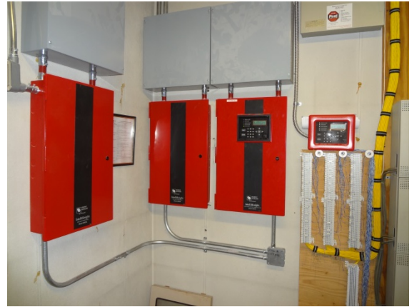
PHOTO #32: CAMPUS FIRE ALARM SYSTEM (HONEYWELL)
