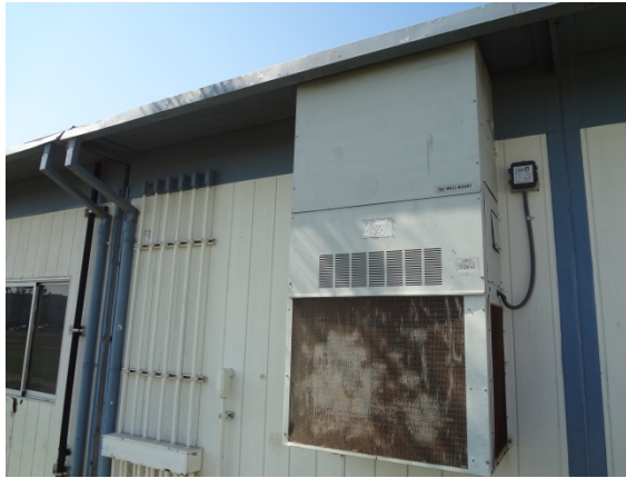
PHOTO #31: PORTABLE BUILDING HEAT PUMP
