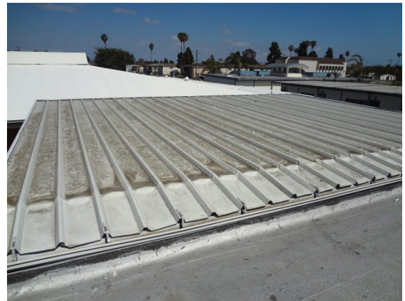
PHOTO #18: LUNCH PAVILION METAL ROOF
