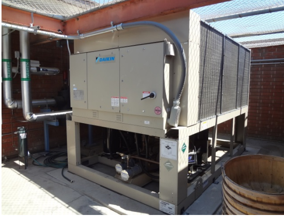
PHOTO #25: MAIN BUILDING AIR COOLED CHILLER
