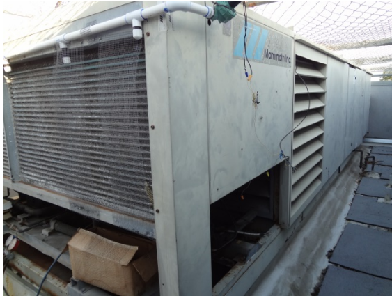
Photo #49: Mammoth Rooftop Unit
