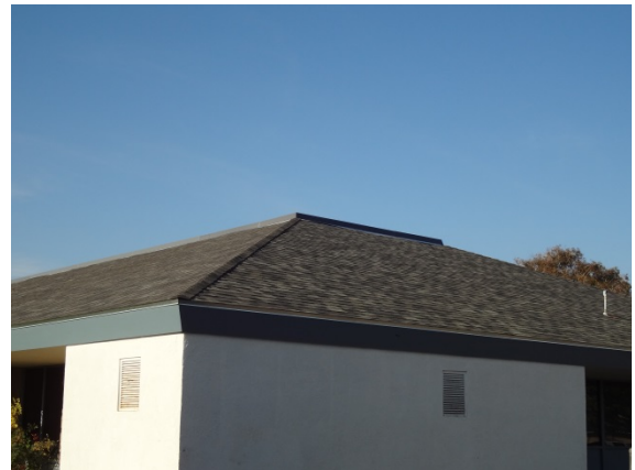
Photo #30: Asphalt Shingle Roof
