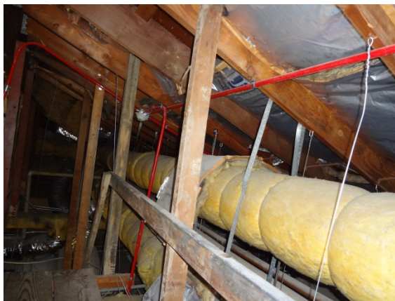
Photo #41: Building A-D Attic
