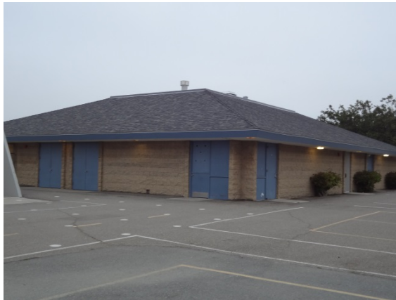
Photo #9: Building C Elevation
