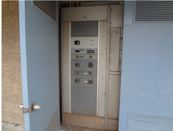
Photo #55: Main Switchboard
