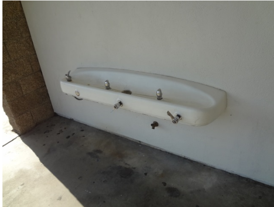
Photo #43: Exterior Drinking Fountain
