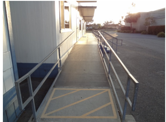
Photo #28: Portable Building Metal Ramp
