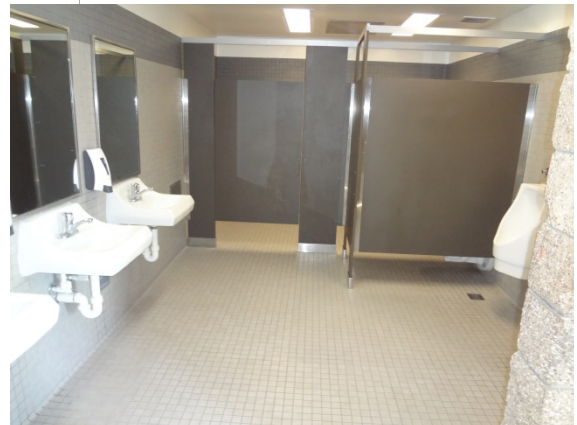
Photo #46: Restroom Fixtures
