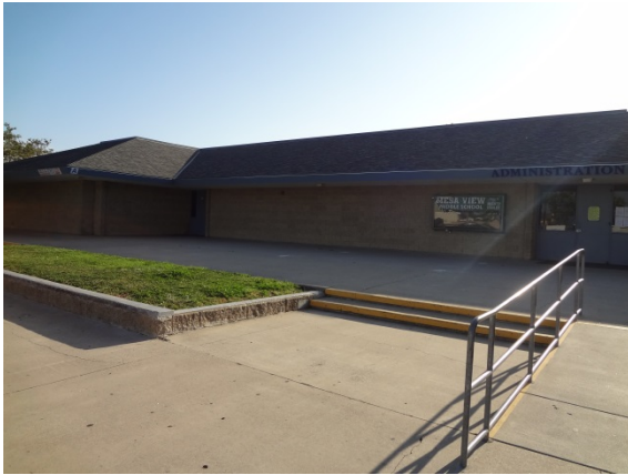
Photo #1: Administration Building Front Elevation
