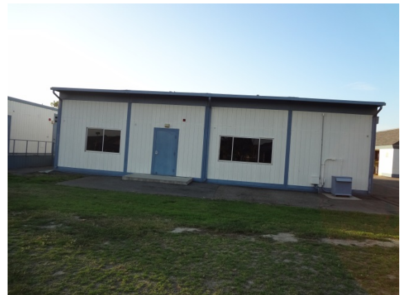
Photo #6: PAC Rear Elevation
