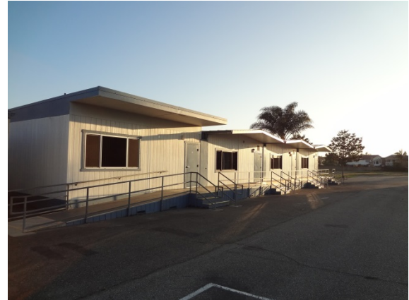
Photo #8: P1-P4 Elevation
