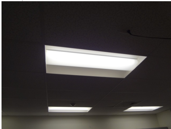
Photo #45: Fluorescent Interior Light Fixture
