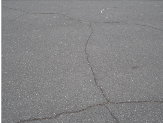
Photo #25: Minor Cracking Throughout Asphalt Playground
