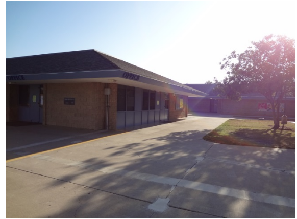
Photo #2: Administration Building Right Elevation
