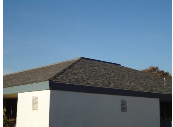
Photo #38: Building A Stucco Finish
