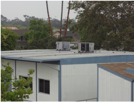
Photo #33: PAC Asphalt Membrane Roof
