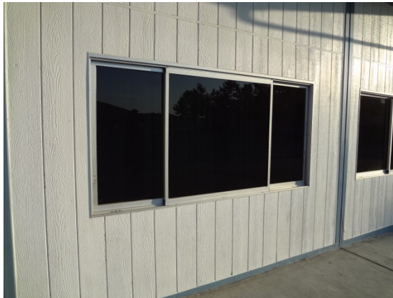
Photo #39: Portable Building Wood Siding
