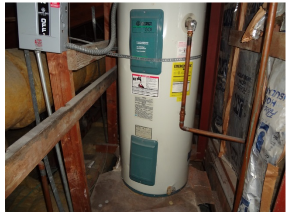
Photo #48: Water Heater
