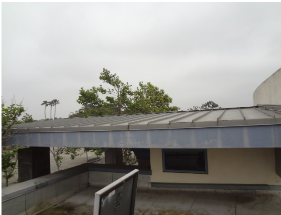
Photo #35: Gym Metal Roof
