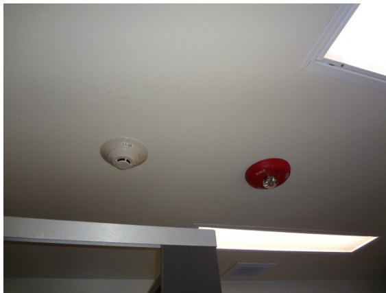
Photo #47: Fire Alarm Devices
