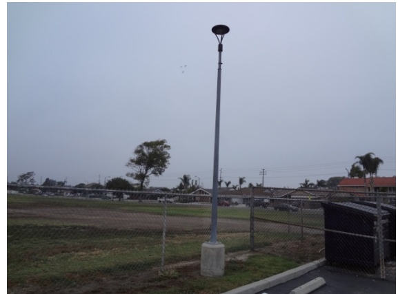
Photo #52: Pole Mounted Exterior Light Fixture
