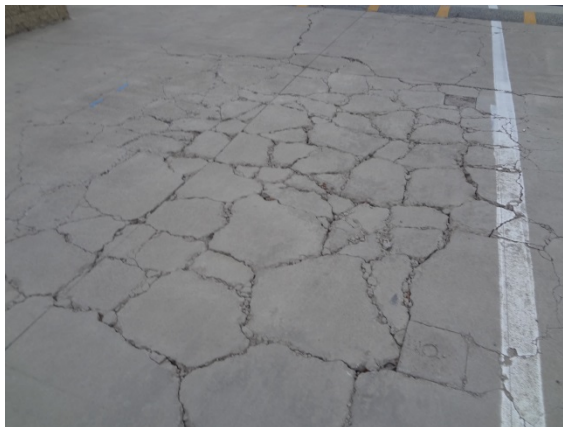
Photo #17: Cracking Section of Concrete Parking Lot
