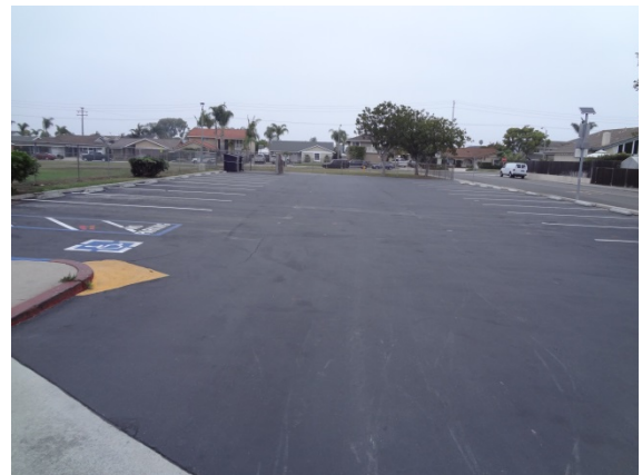
Photo #18: Asphalt Parking Lot North
