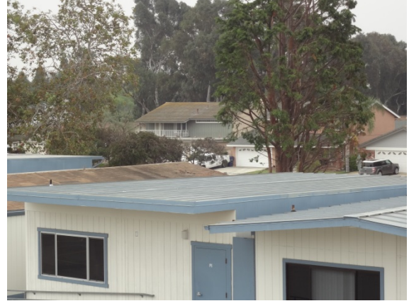
Photo #32: Portable Building Asphalt Membrane Roof
