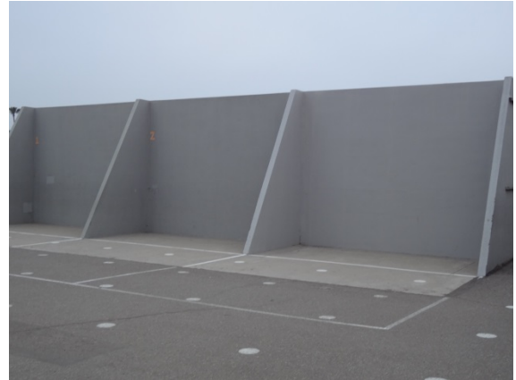
Photo #26: Concrete Backstop
