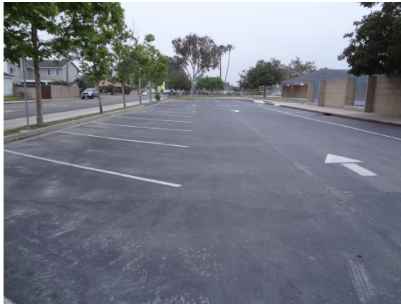
Photo #15: Asphalt Parking Lot South
