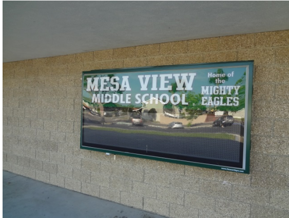
Photo #37: Building A-D CMU Exterior Walls
