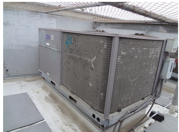
Photo #54: Carrier Packaged Rooftop Unit
