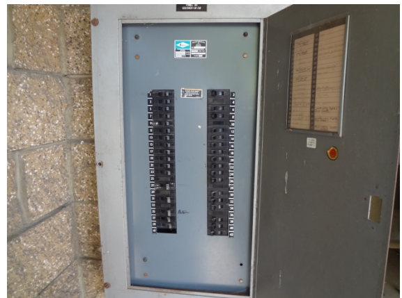
Photo #42: Electrical Panel - Original
