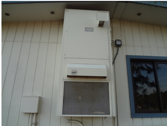
Photo #51: Packaged Heat Pump
