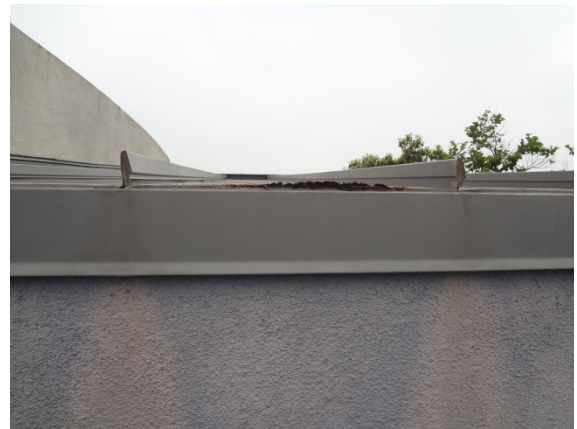
Photo #36: Gym Roof Corroding Edges
