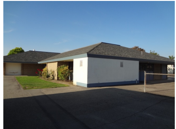
Photo #4: Administration Building Left Elevation
