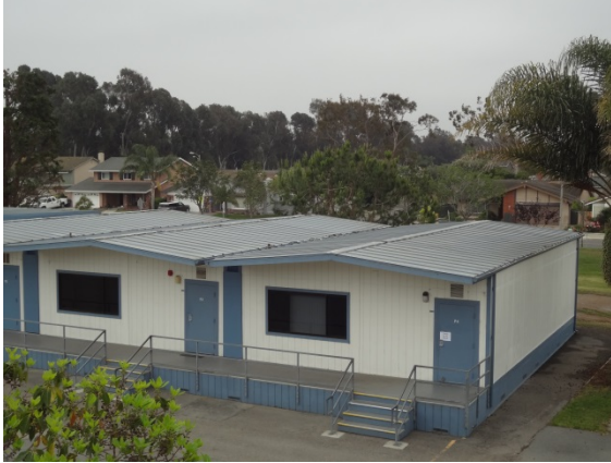
Photo #31: Portable Building Metal Roof
