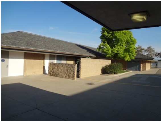
Photo #3: Administration Building Rear Elevation
