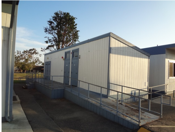
Photo #7: Restroom Building Elevation
