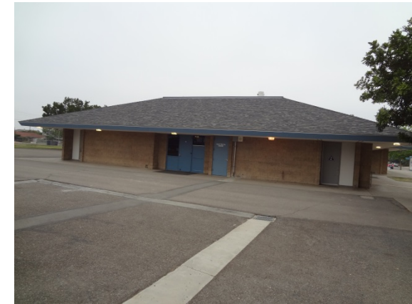
Photo #10: Building D Elevation
