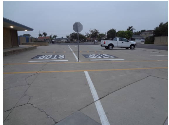
Photo #16: Concrete Parking Lot
