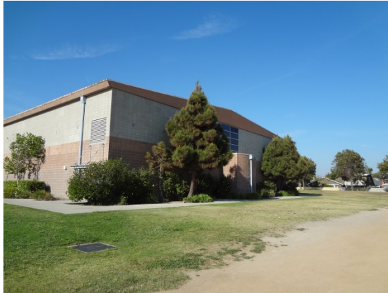
Photo #13: Gym Rear Elevation
