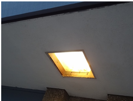
Photo #53: Building Mounted Exterior Light Fixture
