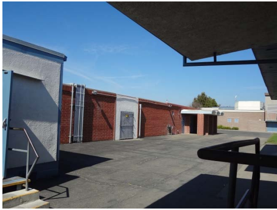
Photo #3: Main Building Rear Elevation
