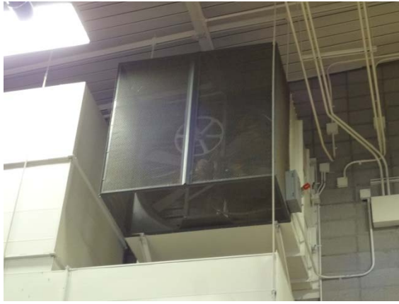
Photo #51: Propeller Exhaust Fan Main Gym
