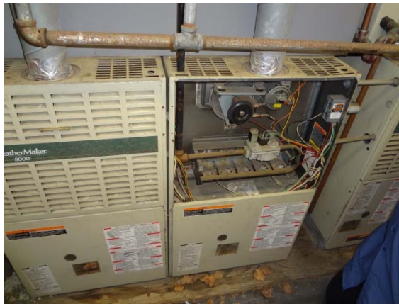
Photo #45: Multipurpose Building Gas Furnaces with DX Cooling
