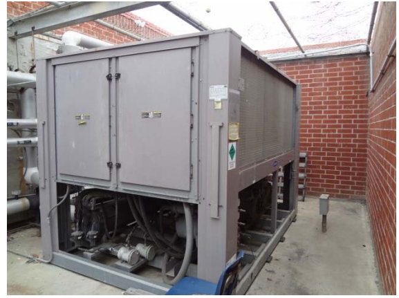
Photo #40: Air Cooled Chiller
