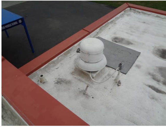
Photo #39: Main Building Roof Mounted Exhaust Fan
