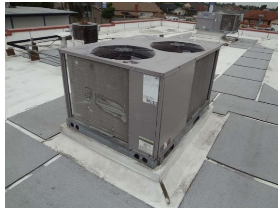
Photo #46: Multipurpose Building Condensing Unit
