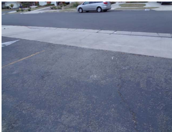
Photo #15: General Cracking Main Lot
