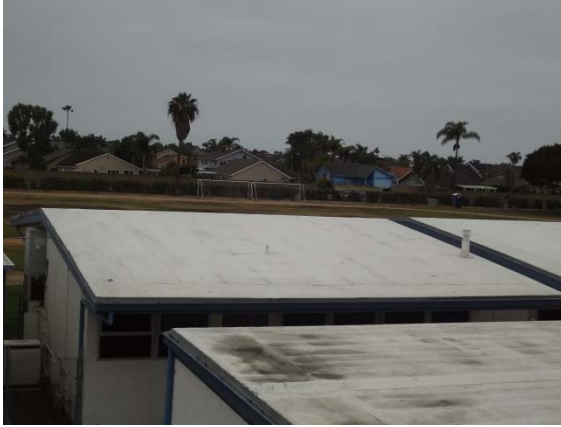
Photo #25: Portable Building Asphalt Membrane Roof
