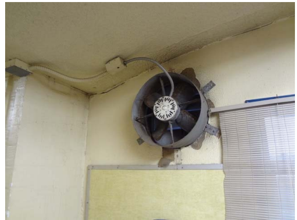
Photo #36: Concession Exhaust Fan
