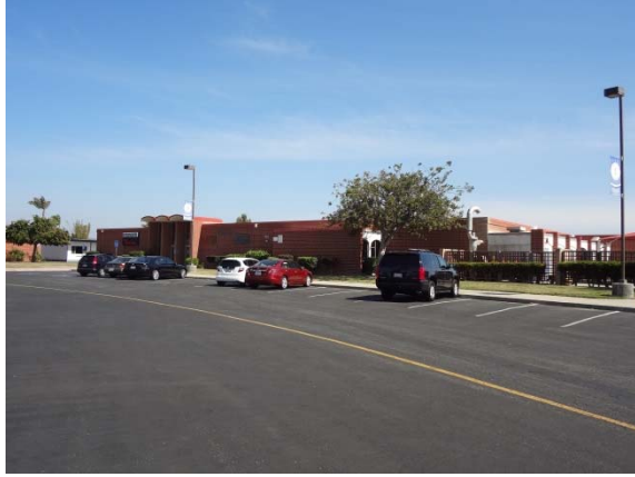
Photo #1: Main Building Front Elevation
