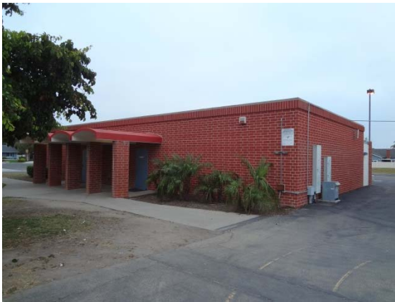
Photo #27: Brick Façade (Main, Library, Multipurpose)
