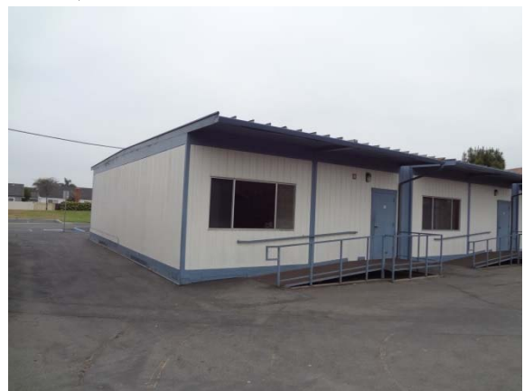
Photo #6: Portable Classroom Front Elevation
