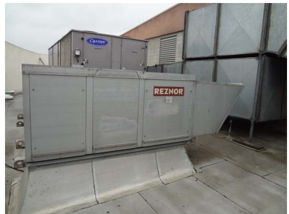
Photo #48: Gym Gas Fired Rooftop Unit
