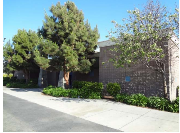
Photo #8: Gym Building Front Elevation
