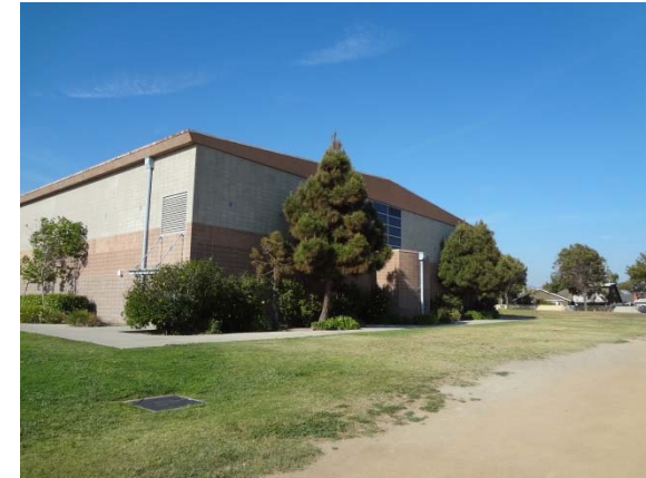
Photo #10: Gym Building Rear Elevation
