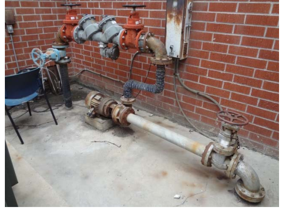
Photo #44: Irrigation Pump and Backflow Preventer
