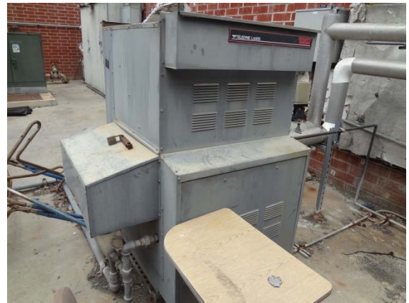
Photo #42: Heating Water Boiler
