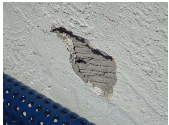
Photo #30: Damaged Stucco Finish at Portable Building
