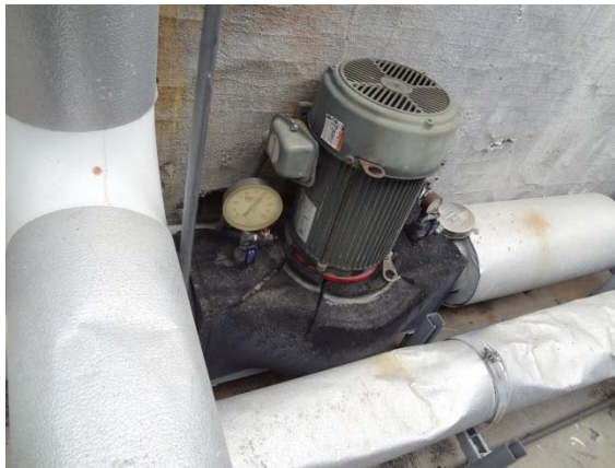
Photo #41: Dual Temperature Circulation Pump
