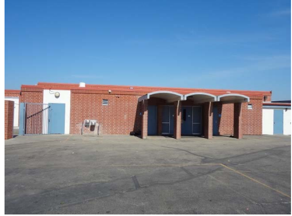
Photo #2: Main Building Right Elevation
