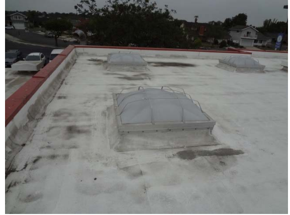
Photo #26: Main Building Dome Style Skylight
