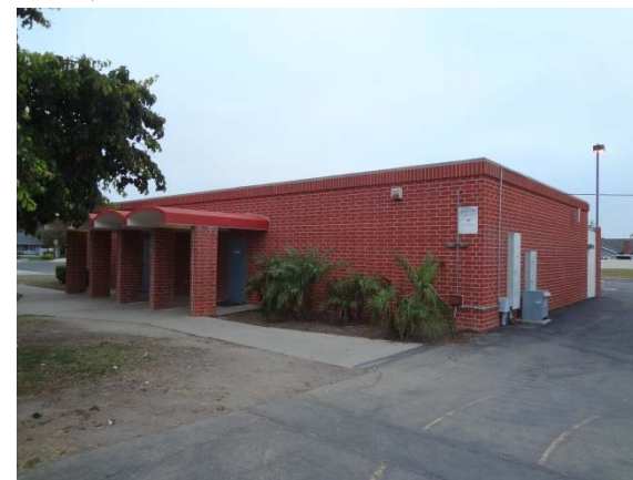
Photo #5: Library Building Front Elevation
