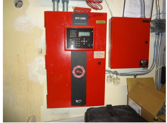
Photo #38: Fire Alarm Panel
