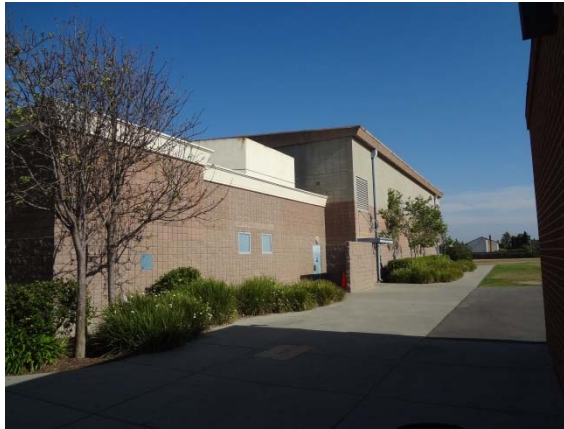
Photo #9: Gym Building Right Elevation
