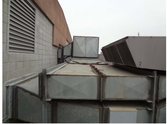
Photo #50: Deteriorating Roof Ductwork at Gym
