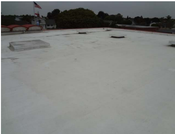
Photo #23: Main Roof Asphalt Membrane
