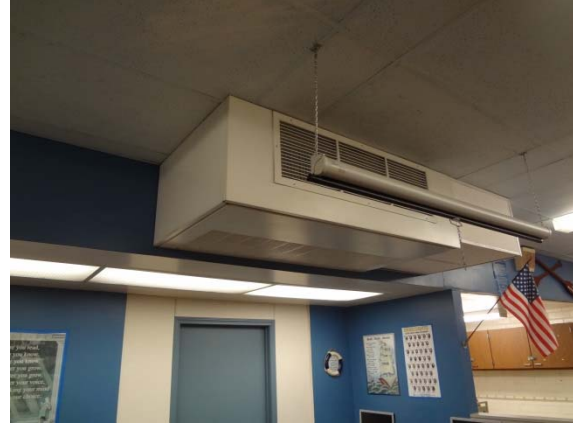
Photo #32: 2-Pipe Fan Coil Unit
