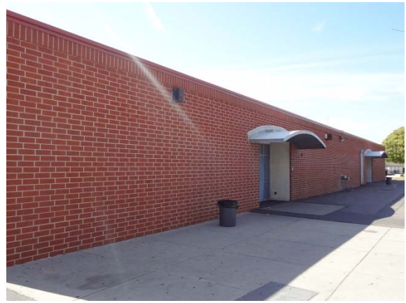
Photo #4: Main Building Left Elevation
