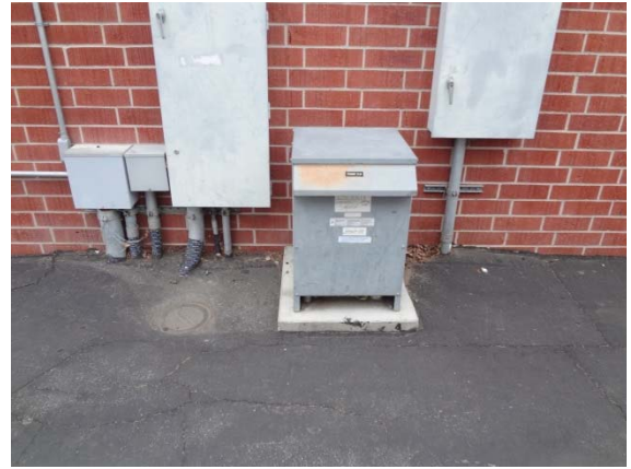
Photo #34: Exterior Pad Mounted Transformer
