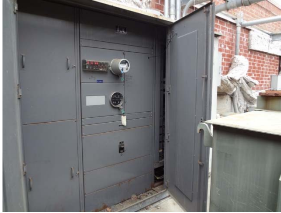
Photo #43: Main Switchboard
