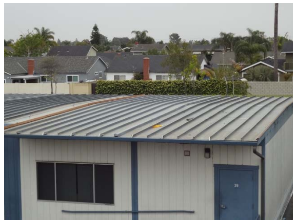
Photo #24: Portable Building Metal Roof
