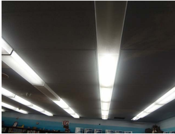
Photo #33: T-8 Fluorescent Light Fixtures
