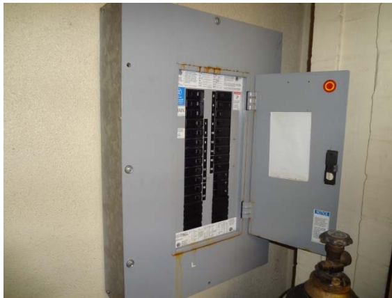
Photo #35: Electrical Panel
