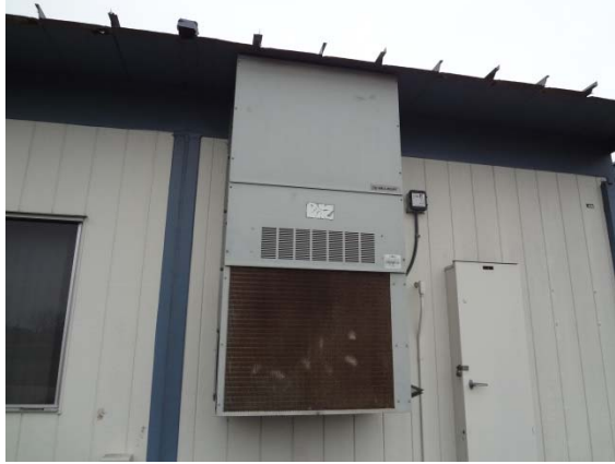
Photo #37: Portable Building Packaged Heat Pump
