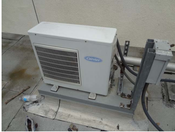
Photo #49: Ductless Split System Condensing Unit
