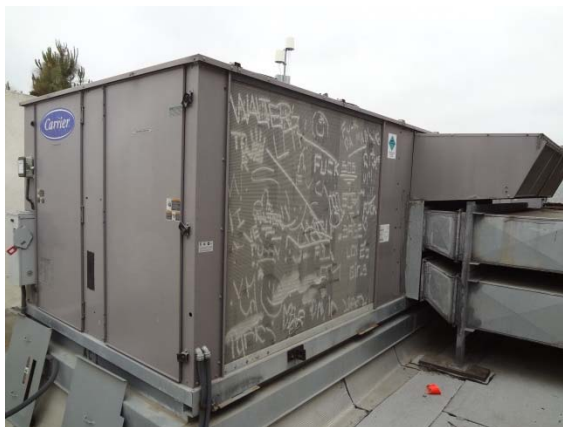
Photo #47: Gym Packaged Rooftop Unit
