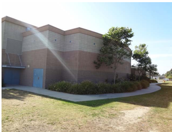
Photo #11: Gym Building Left Elevation
