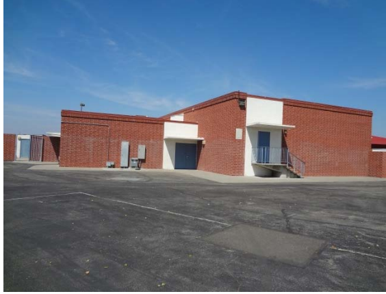
Photo #7: Multipurpose Building Rear Elevation
