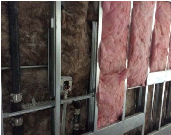
Photo #39: Fiberglass insulation
