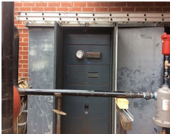
Photo #27: Main switchgear
