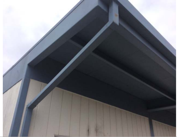
Photo #20: Soffit, gutter and downspout at portables
