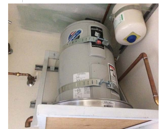
Photo #24: Electric water heater
