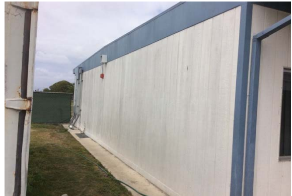
Photo #4: Side view of a portable building
