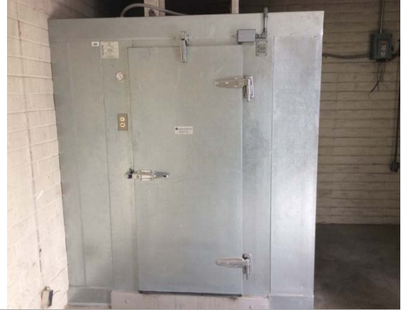
Photo #32: Walk-in freezer
