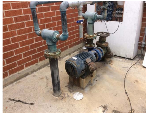
Photo #26: Irrigation pump
