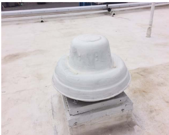
Photo #23: Exhaust fan
