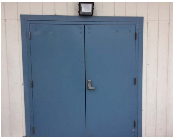
Photo #41: Double metal exterior door
