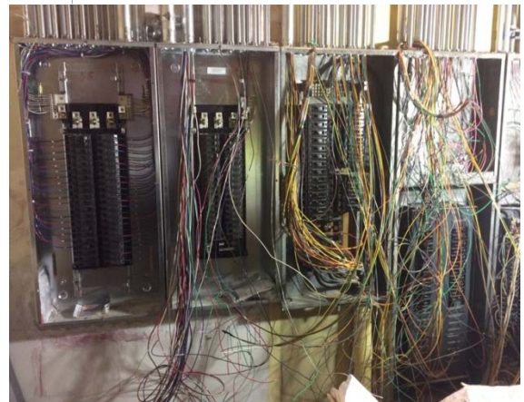
Photo #28: Newly installed panel boxes
