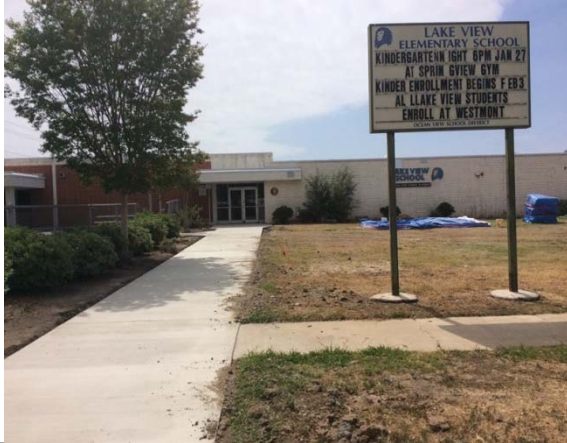
Photo #1: Front elevation of Main Building
