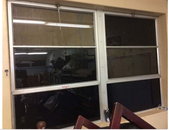
Photo #44: Aluminum-framed hopper window
