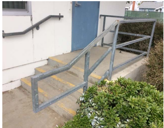
Photo #22: Concrete stairs with metal rails
