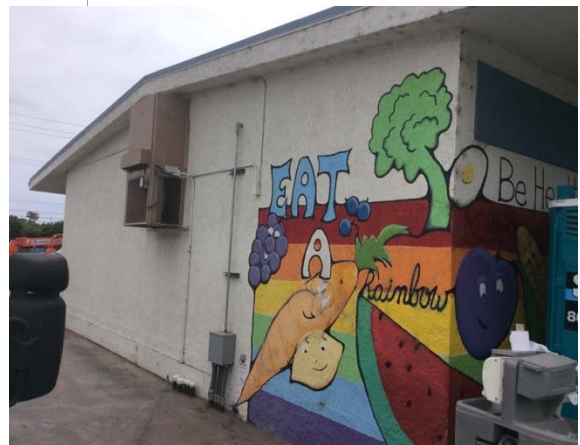
Photo #6: Side view of Building 19
