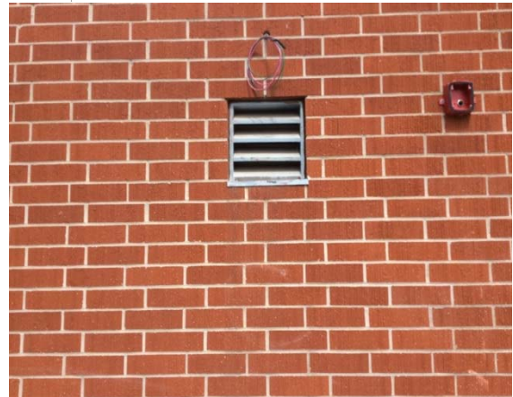
Photo #34: Wall ventilation
