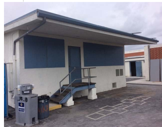
Photo #5: Front view of Building 19
