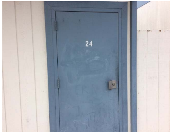
Photo #40: Single metal exterior door
