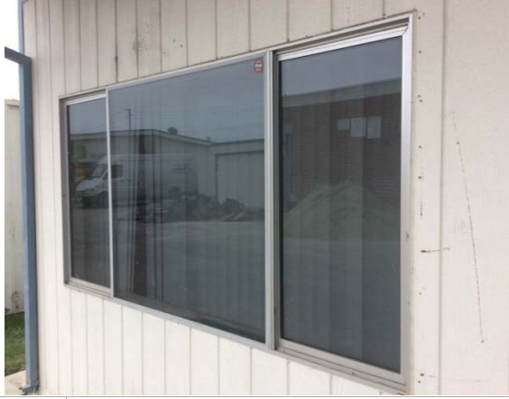
Photo #43: Aluminum-framed sliding window
