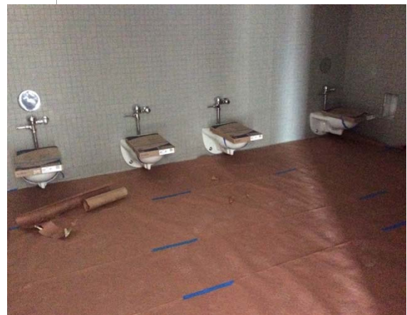
Photo #36: Water closets
