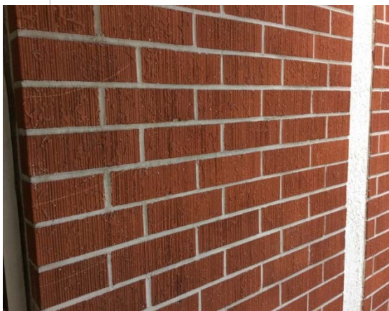
Photo #17: Exterior CMU wall at Main Building
