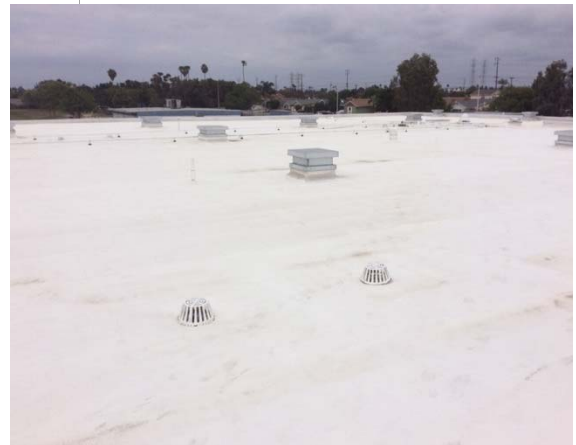
Photo #16: Overview of roofing at Main Building
