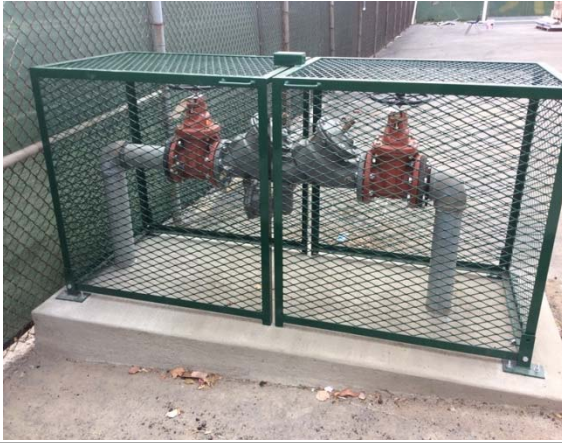
Photo #31: Backflow preventer
