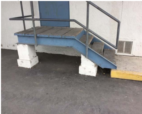
Photo #21: Steel framed with wood treads stairs
