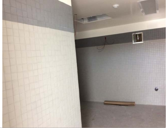
Photo #38: Ceramic wall tiles in bathroom
