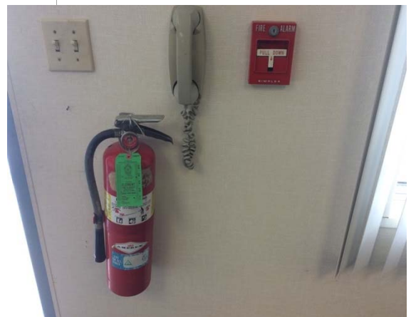
Photo #30: Fire extinguisher and pull station
