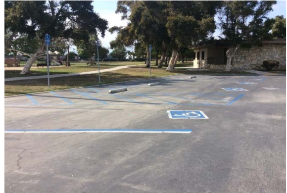
Photo #8: Parking lot with ADA spaces
