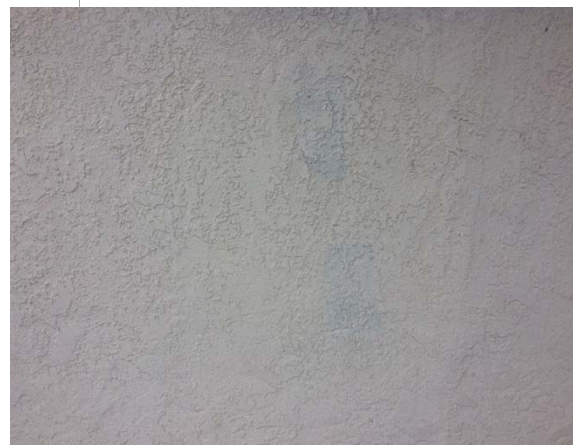
Photo #18: Stucco wall at Building 19
