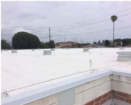
Photo #15: Overview of roofing at Main Building
