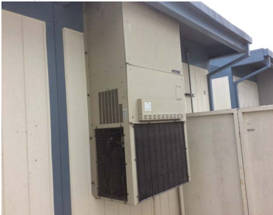
Photo #33: Wall-mounted package heat pump
