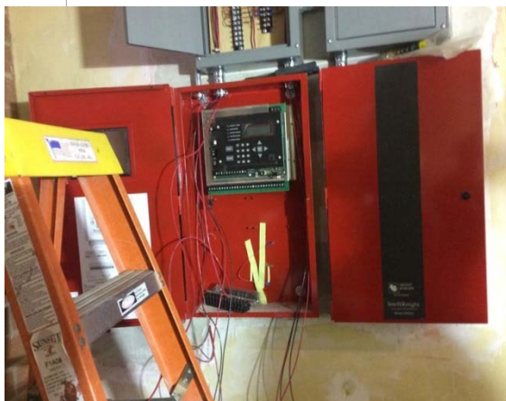
Photo #29: Fire alarm control panel
