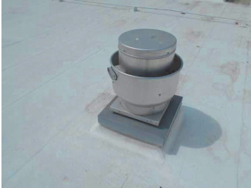
PHOTO #49: ROOFTOP POWERED EXHAUST FAN
