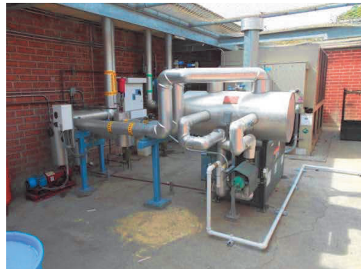
PHOTO #40: HOT WATER BOILER
