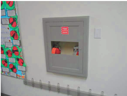
PHOTO #45: FIRE EXTINGUISHER CABINET
