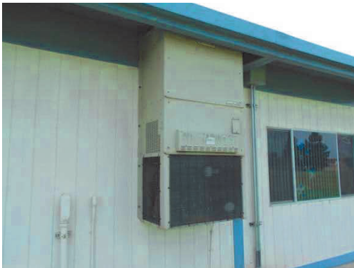
PHOTO #39: WALL MOUNTED HEAT PUMP
