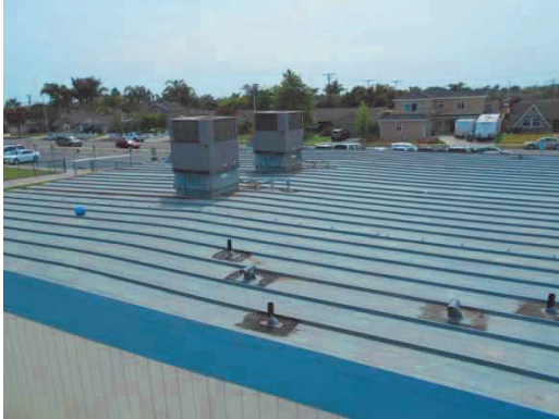
PHOTO #31: PORTABLE BUILDING SHEET METAL ROOF
