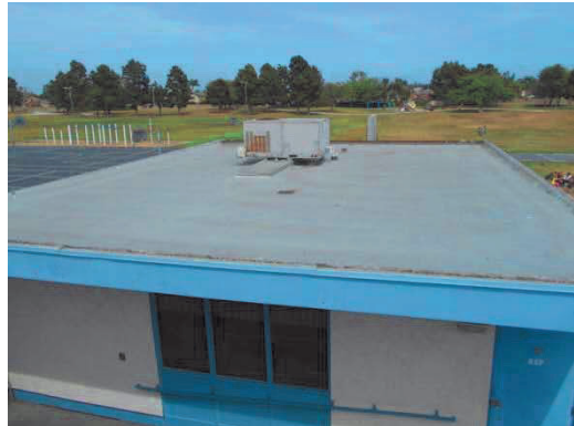
PHOTO #28: PORTABLE BUILDING BUILT-UP ROOF
