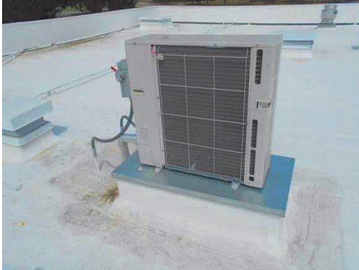
PHOTO #37: DUCTLESS SPLIT SYSTEM CONDENSING UNIT
