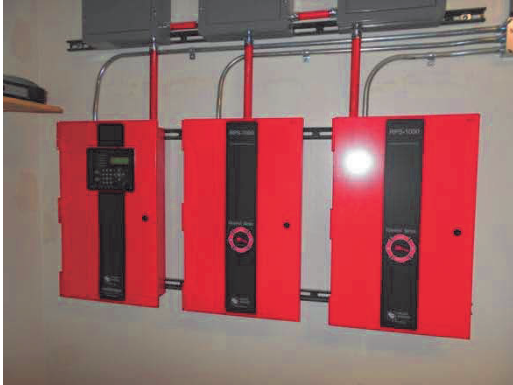
PHOTO #43: CENTRAL ALARM PANEL
