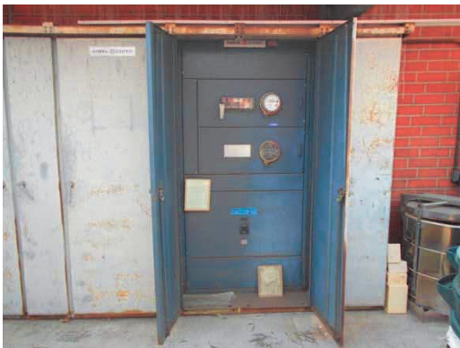
PHOTO #47: ELECTRIC MAIN SWITCHGEAR
