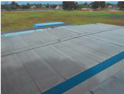
PHOTO #29: PORTABLE BUILDING BUILT-UP ROOF
