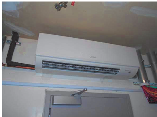
PHOTO #36: DUCTLESS SPLIT SYSTEM INTERIOR FAN
