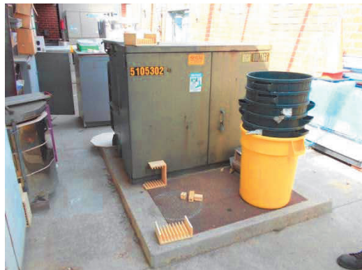
PHOTO #48: PAD MOUNTED TRANSFORMER
