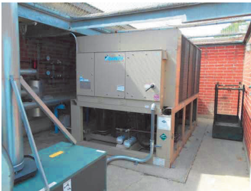
PHOTO #41: AIR COOLED CHILLER
