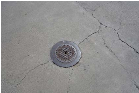
Photo #59: Drain in Dumpster Area
