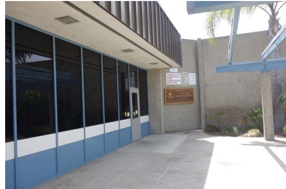
Photo #10: Front Entrance Soffit
