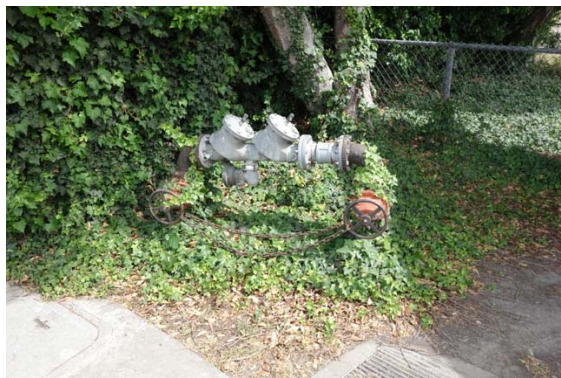
Photo #53: Domestic Water Supply Shut-off and Backflow Preventer
