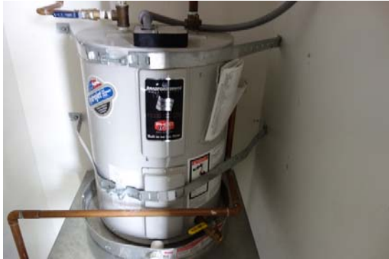
Photo #25: Electric 20 Gal Domestic HW
