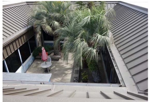
Photo #40: Soffit and Gutter View
