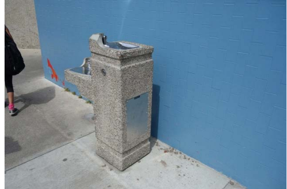
Photo #26: Outside Drinking Fountain
