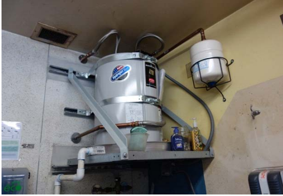
Photo #19: Mechanical Room NW Area
