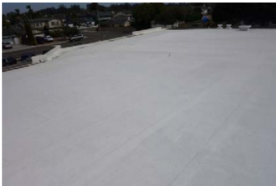
Photo #35: Builtup Roof with Elastomeric Coating
