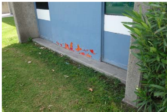
Photo #11: Exterior Wood Panel Damage
