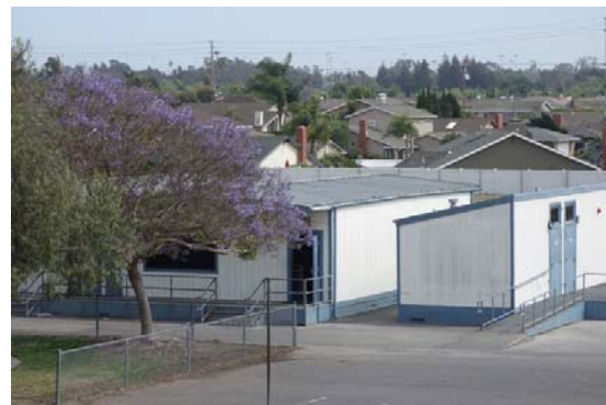
Photo #36: Portable Roof View
