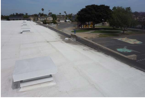
Photo #37: South View and Roof Drain
