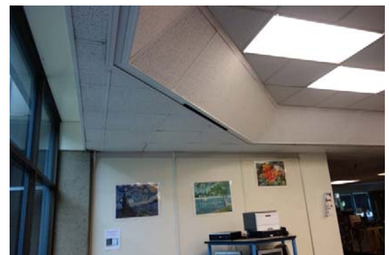
Photo #30: Classroom Ceiling
