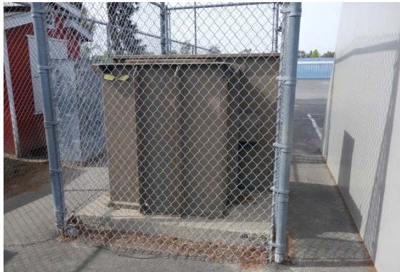
Photo #57: Main Site Transformer
