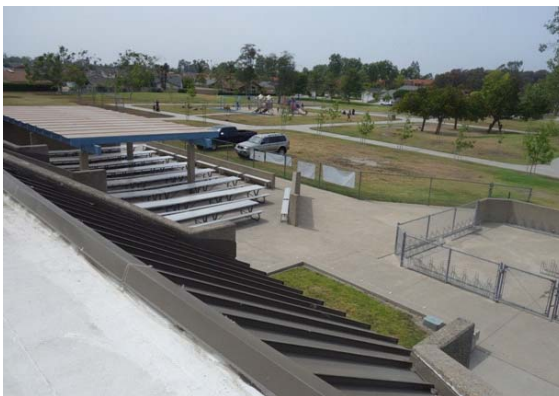
Photo #41: North View and Chain Link Fence
