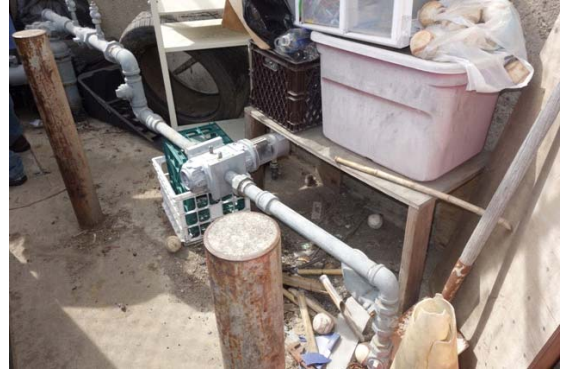
Photo #56: Main Gas Shutoff
