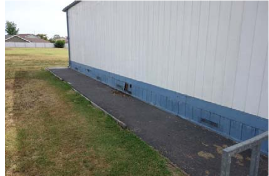
Photo #50: Portable Wooden Panel Damage
