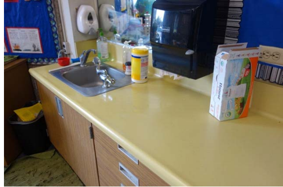
Photo #32: Classroom Sink and Faucets
