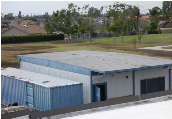
Photo #39: Portable with Asphalt Roof
