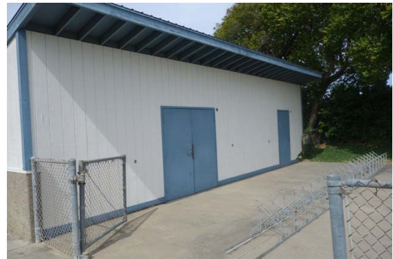
Photo #52: Maintenance Building
