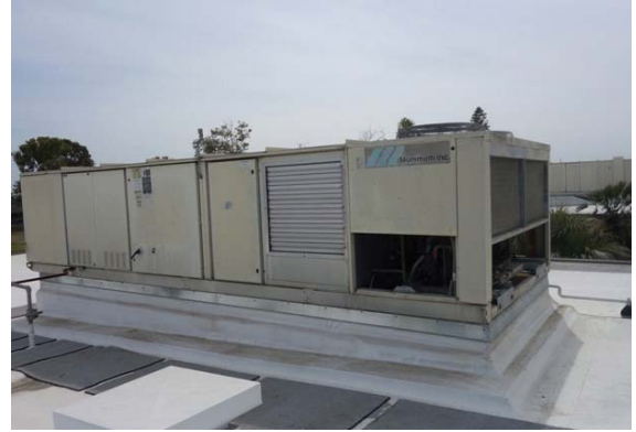
Photo #38: 25 Ton Mammoth Heating and AC Package Unit
