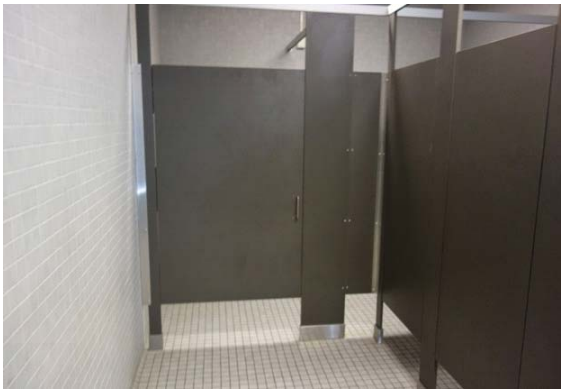
Photo #21: New RR Partitions
