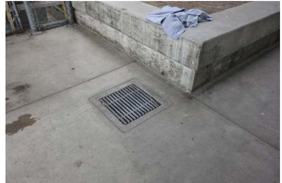
Photo #28: Outside Drain
