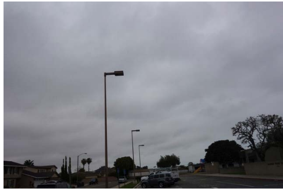
Photo #58: Site Lighting
