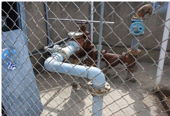
Photo #51: Irrigation Supply Valve
