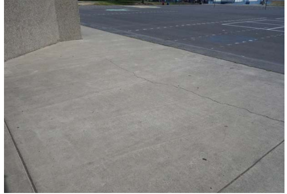
Photo #20: Concrete Sidewalk
