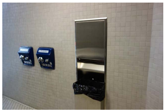
Photo #22: RR Wall detail
