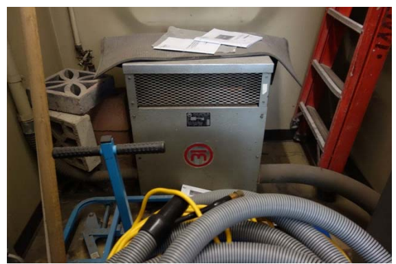
Photo #18: Stepdown Transformer
