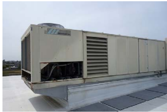
Photo #34: 20 Ton Mammoth Heating and AC Package Unit
