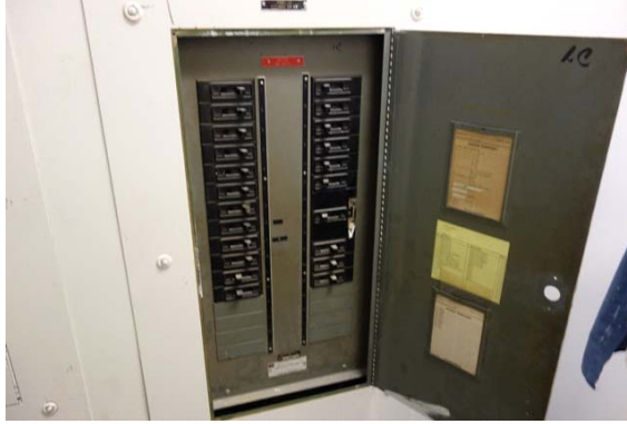
Photo #55: Original Electrical Breaker Panel
