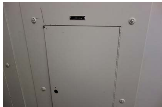
Photo #54: Electrical Breaker Panel
