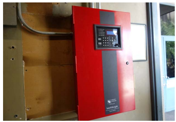
Photo #16: Fire Panel in Custodian Office
