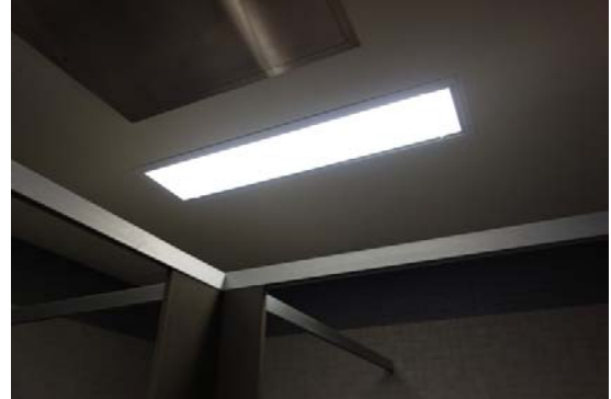
Photo #8: Staff RR Lighting
