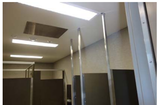
Photo #24: New RR Ceiling Detail
