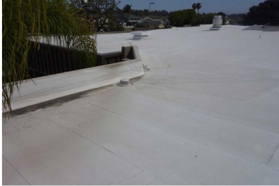
Photo #43: Roof and Roof Drain
