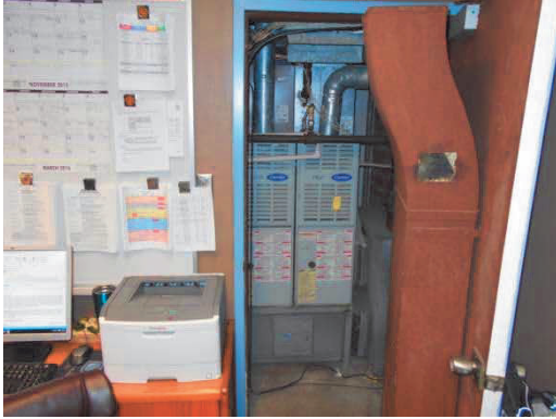
PHOTO #31: GAS FURNACE
