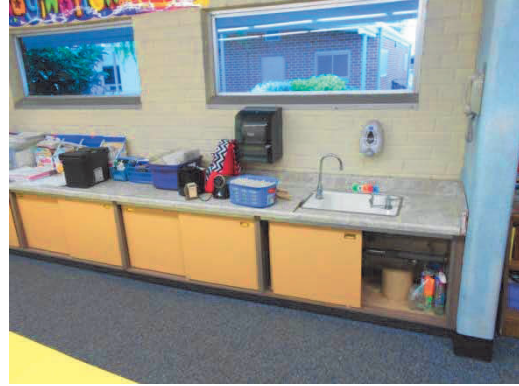
PHOTO #56: CASEWORK INSIDE CLASSROOM
