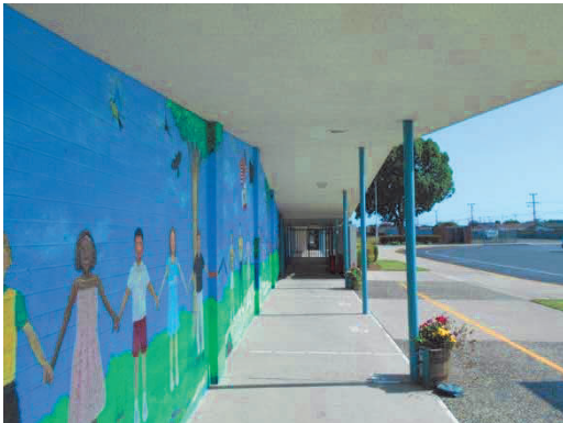
PHOTO #29: COVERED WALKWAY
