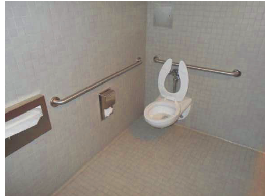
PHOTO #52: ACCESSIBLE RESTROOM
