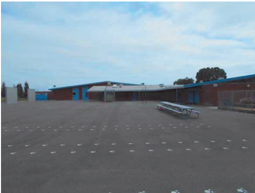
PHOTO #3: WEST ELEVATION
