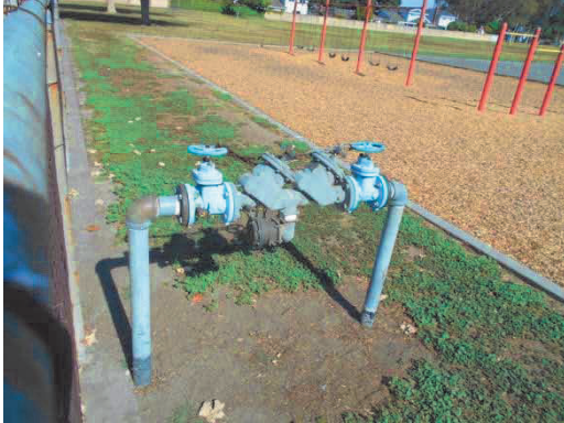
PHOTO #43: BACKFLOW PREVENTER
