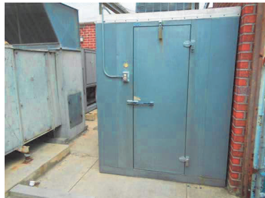
PHOTO #48: WALK-IN FREEZER
