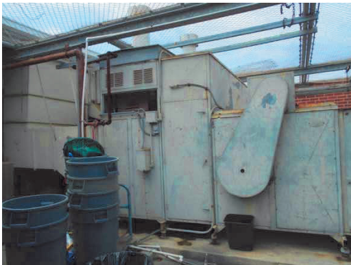
PHOTO #39: GROUND MOUNTED PACKAGED AIR HANDLING UNIT
