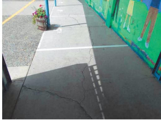
PHOTO #20: CONCRETE SIDEWALK
