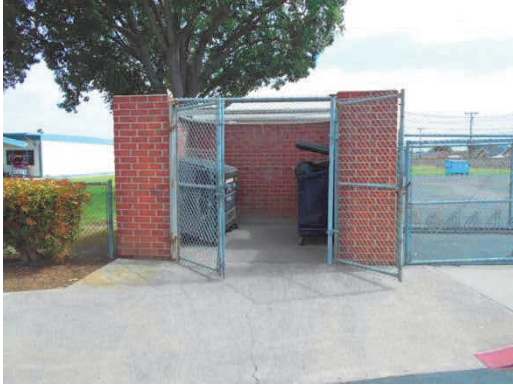
PHOTO #19: TRASH ENCLOSURE
