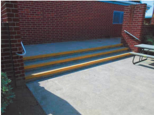
PHOTO #21: SITE CONCRETE STAIR
