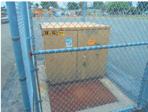
PHOTO #41: PAD MOUNTED TRANSFORMER
