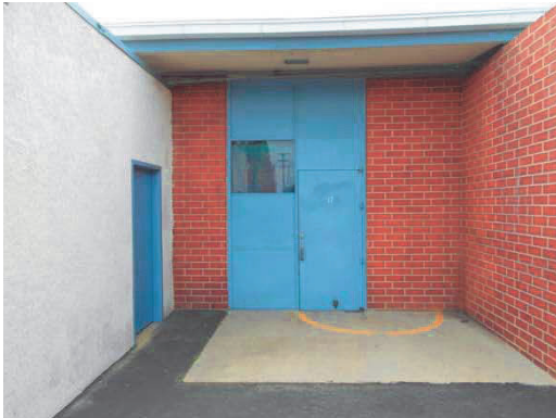
PHOTO #27: SECONDARY ENTRANCE
