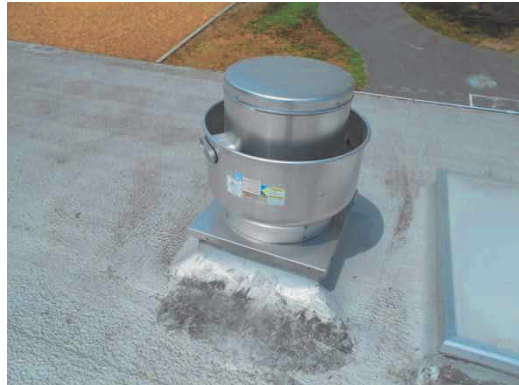
PHOTO #34: POWER VENT
