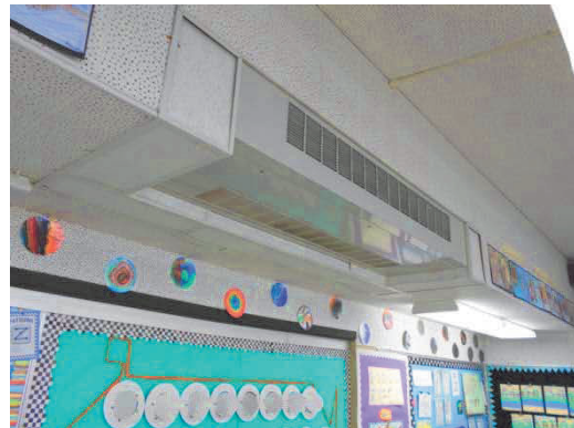
PHOTO #40: FAN COIL UNIT
