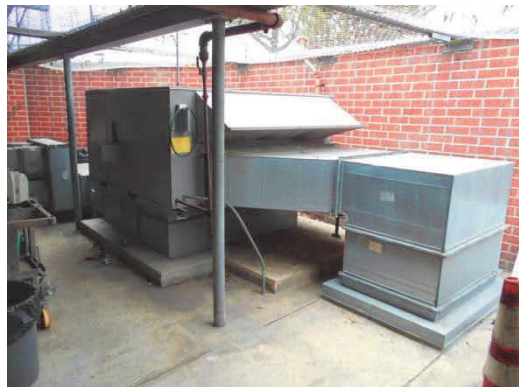
PHOTO #36: GROUND MOUNTED PACKAGED AIR HANDLING UNIT
