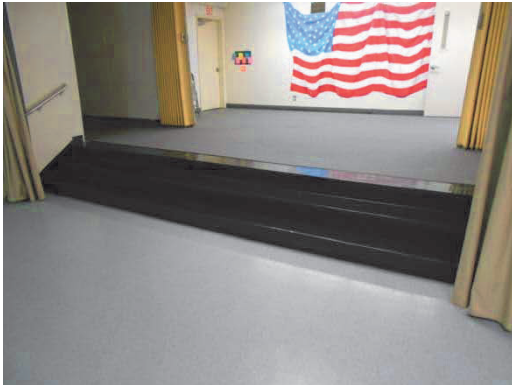
PHOTO #57: INTERIOR STAIR
