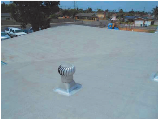
PHOTO #33: GRAVITY VENT
