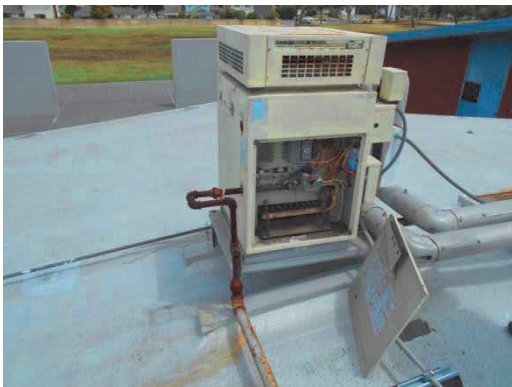
PHOTO #35: ROOFTOP BOILER
