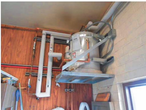
PHOTO #47: DOMESTIC WATER HEATER
