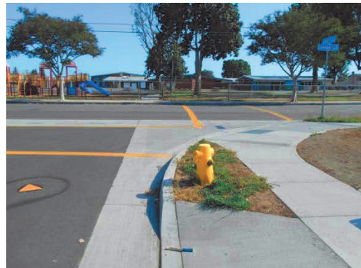
PHOTO #46: FIRE HYDRANT
