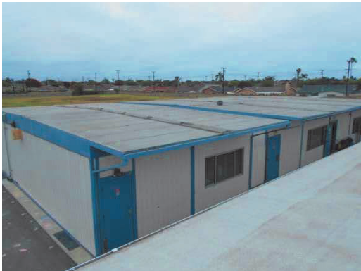
PHOTO #23: PORTABLE BUILDING BUILT-UP ROOF
