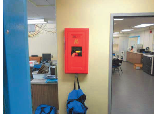
PHOTO #44: CENTRAL FIRE CONTROL PANEL
