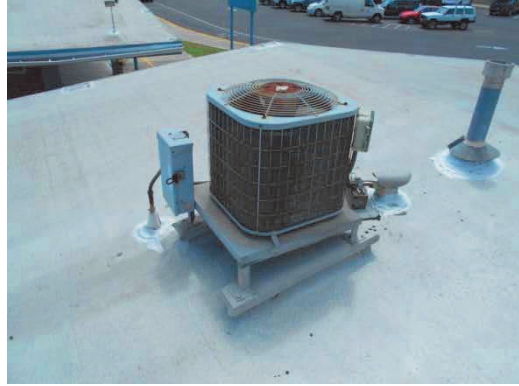
PHOTO #32: ROOFTOP CONDENSING UNIT
