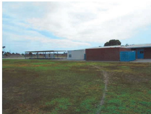
PHOTO #5: NORTH ELEVATION
