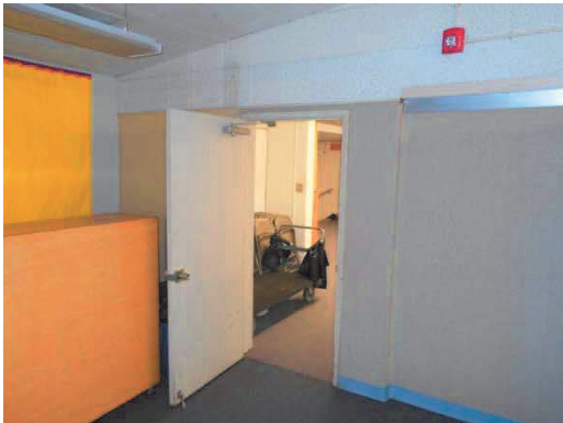
PHOTO #53: INTERIOR WOOD DOOR
