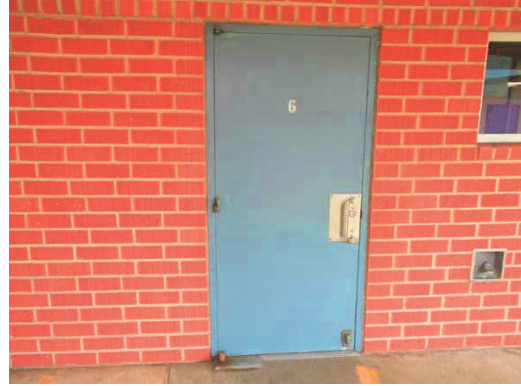
PHOTO #26: STEEL SERVICE DOOR
