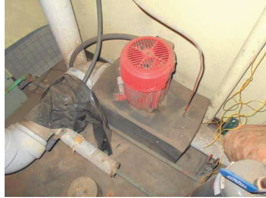
PHOTO #38: WATER CIRCULATION PUMP
