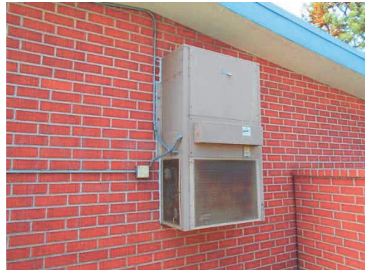
PHOTO #30: PACKAGE HEAT PUMP
