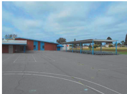
PHOTO #6: EAST ELEVATION
