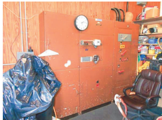
PHOTO #42: ELECTRIC MAIN SWITCHGEAR
