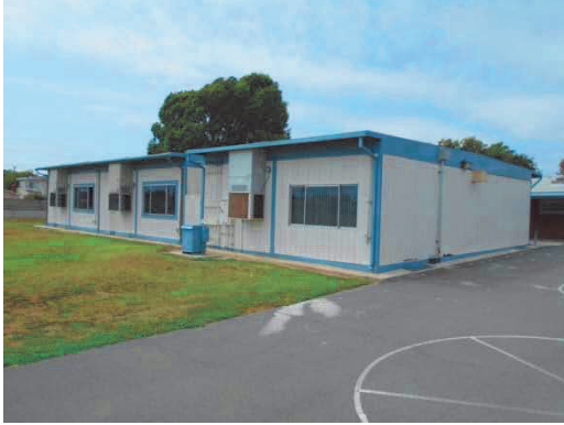
PHOTO #7: PORTABLE BUILDING ELEVATION
