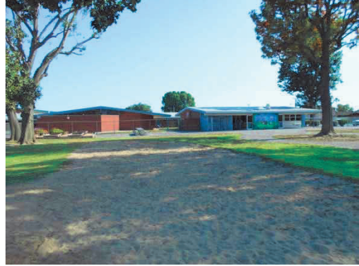
PHOTO #8: WEST ELEVATION
