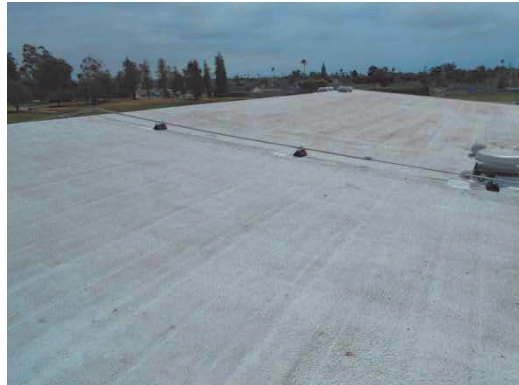
PHOTO #22: MAIN BUILDING BUILT-UP ROOF
